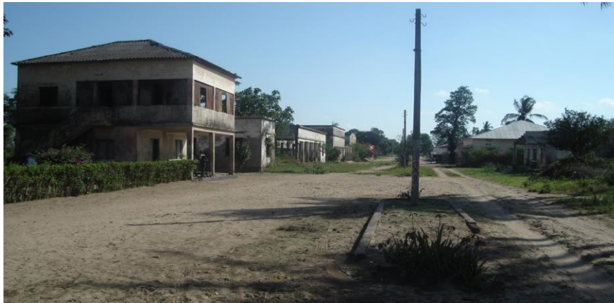
Figure 7.1: Road number 320, Micaúne-Sede village.
