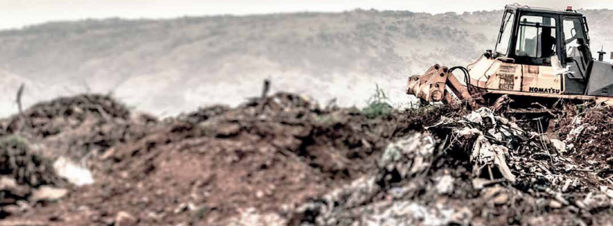
Figure 69 - Earth moving equipment shaping the waste (Author 2016)
