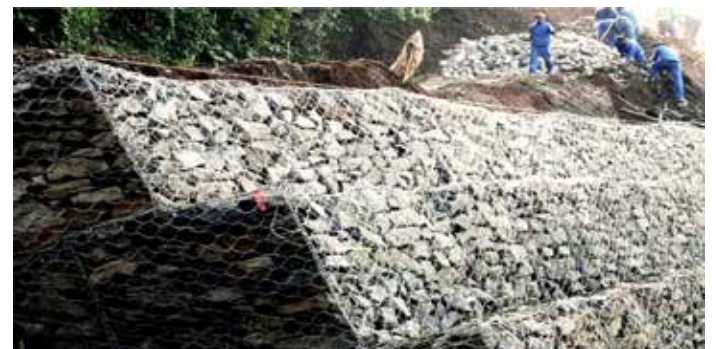
Figure 114 - Example of gabions used to reinforce steep slope and prevent erosion
