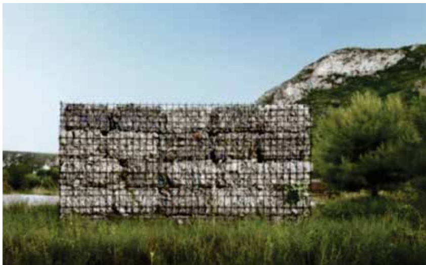
Figure 65 - Gabions filled with recycled waste
