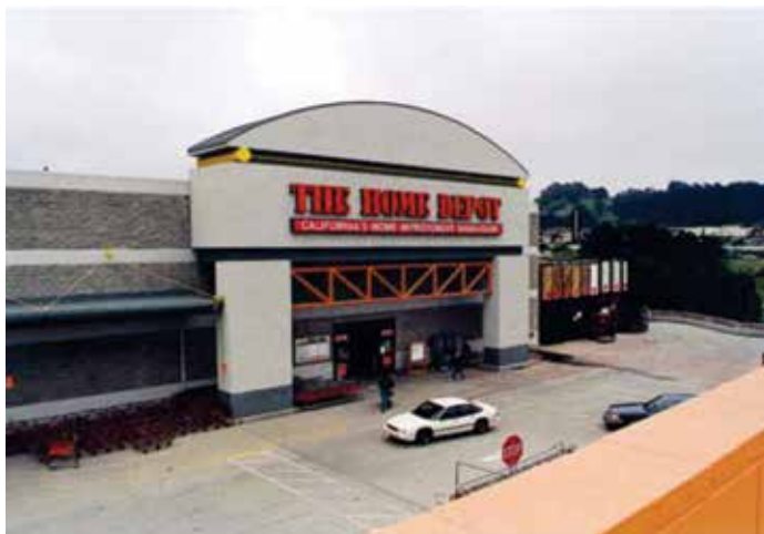
Figure 131 - Retail store on top of a landfill
