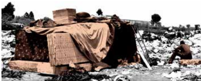
Figure 51 - Here polystyrene is also used as a wall, any large sheets of plastic or carpeting serve a waterproofing layer.
