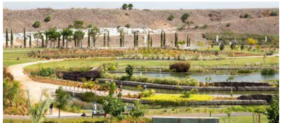
Figure 60 - The park has been designed to include a restaurant and pond on top of the landfill
