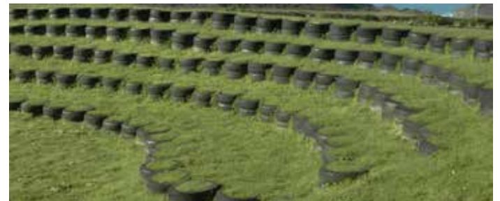
Figure 113- Old tyres stacked to form amphitheater seating & planted with lawn
