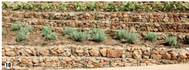
6. Livable terraces are envisioned with each platform being built up with gabion walls filled with material from the landfill.
