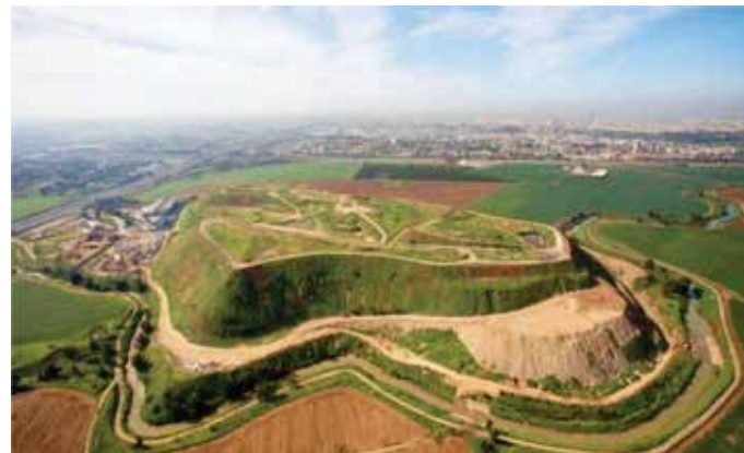
Figure 58 - The Hiriya landfill is over 80m high
