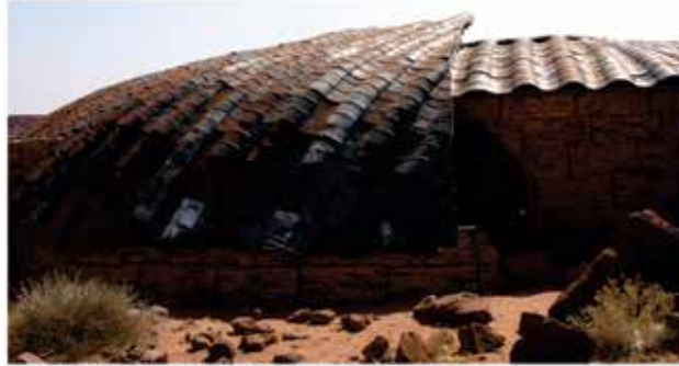
Nina Maritz uses oil drums cut in half to create roofing tiles
