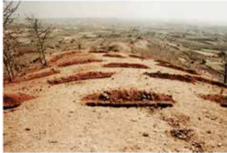
Figure 119 - Trenches dug along contours in a staggered pattern to accumulate soil and create areas for plant growth. (ACF, 2010)
