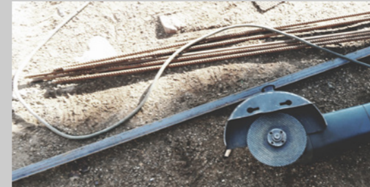
Figure 1.16 Sidewalk working conditions (Author, 2016)
