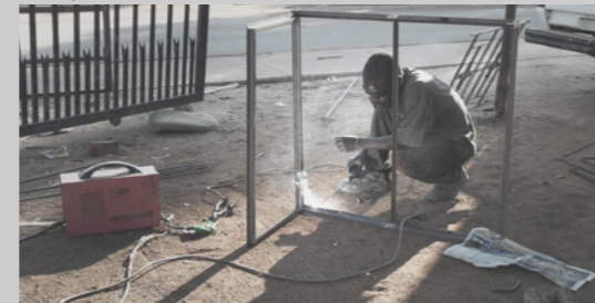
Figure 1.17 Sidewalk as “welding booth”(Author, 2016)
