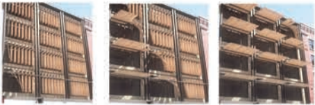
Figure 10.17 Kinetic shading system in different positions (Frearson, 2014)
