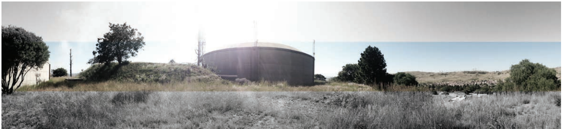
Fig. 71. Atteridgeville Reservoir - north.
