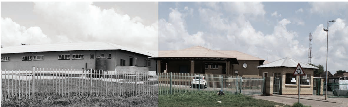
Fig. 43. Atteridgeville Clinic on Mareka street.
