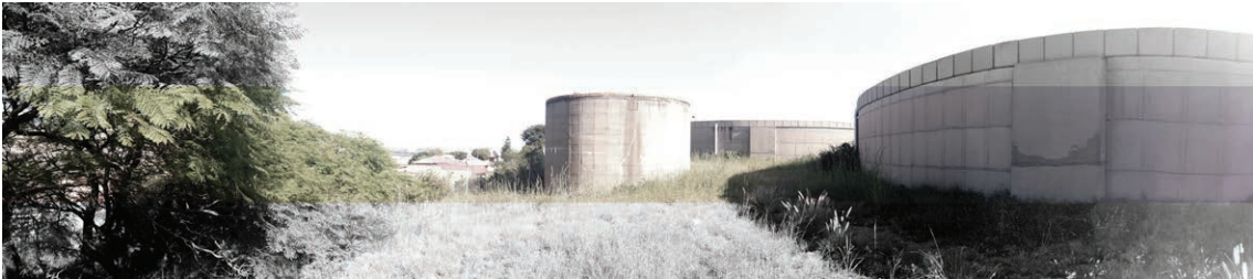
Fig. 67. Atteridgeville Reservoirs - west towards stadium.
