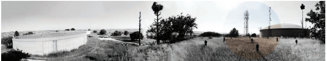
Fig. 70. Atteridgeville Reservoirs - north.
