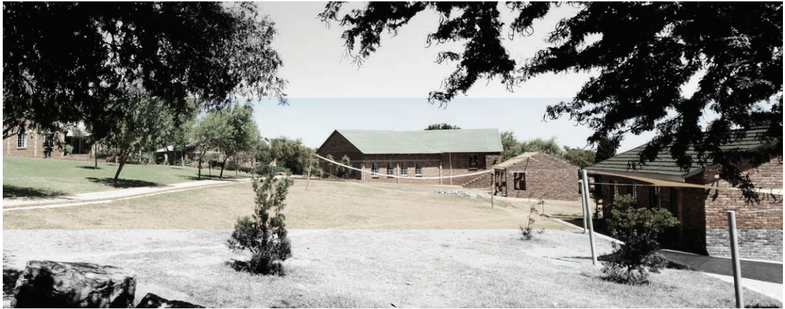
Fig. 65. Classrooms of Holy Trinity High School on Khoza
