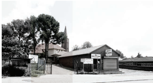
Fig. 51. Church and drycleaners on Seeiso street.
