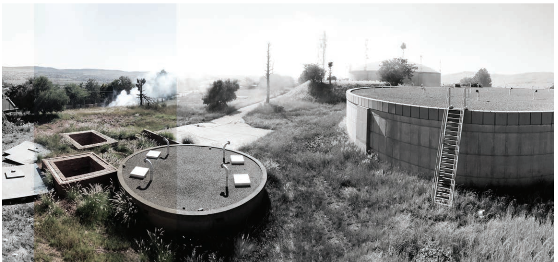
Fig. 72. Atteridgeville Reservoir - east.
