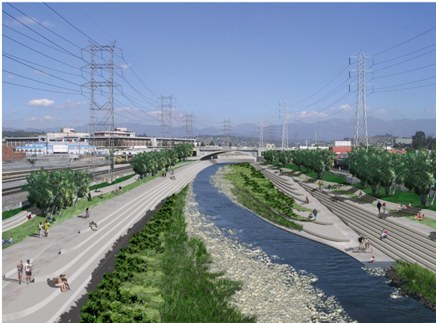
Figure 2.27. Los Angeles River Restoration. www.asla.org. 2013.
