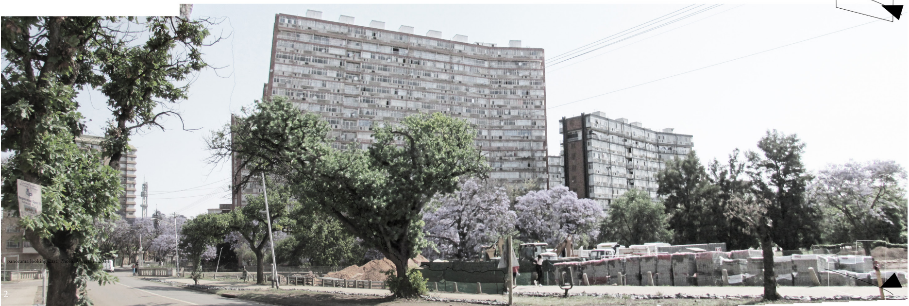
Fig 3.21 Current condition of site, looking South. (Author, October 2016)
