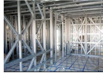
Figure 8.14: Light steel framing
