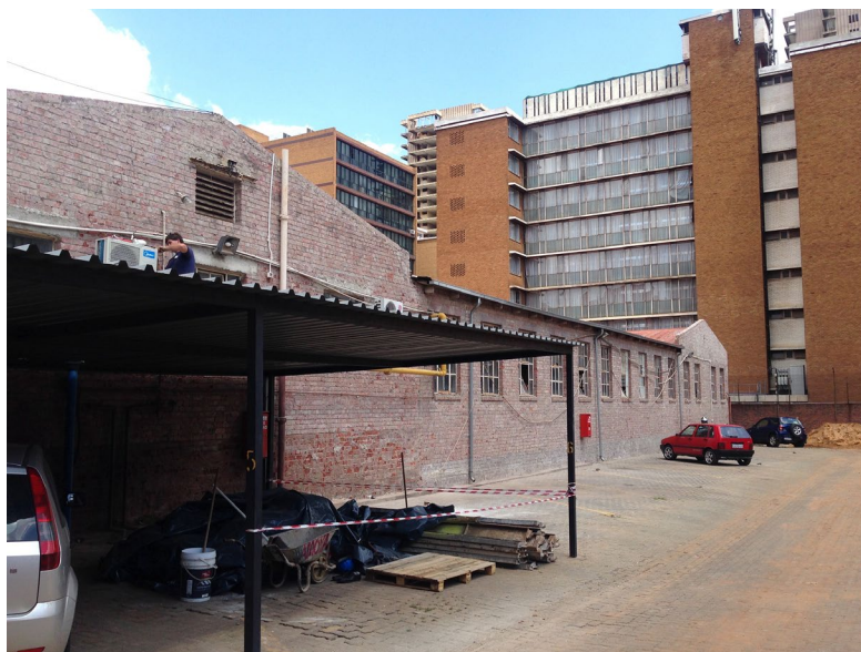
Figure 4.15: Maintenance offices building, Huis Davidtz in the background
