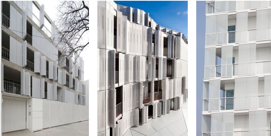
Figure 6.8: Adjustable exterior screening
