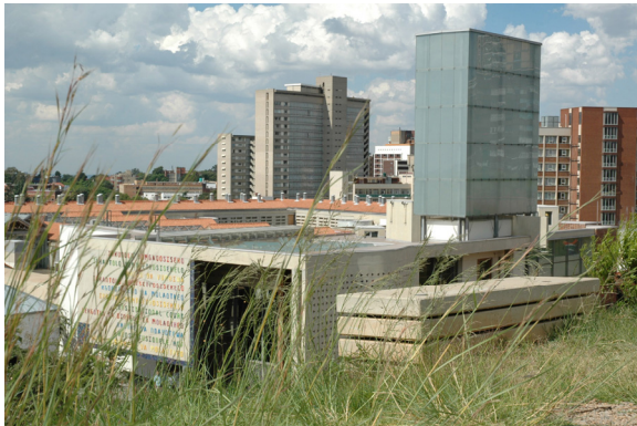
FIGURE 9: The New Constitutional Court of South Africa as catalyst and bridge between Hillbrow and Braamfontein. OMM Design Workshop and Urban Solutions 2004.
