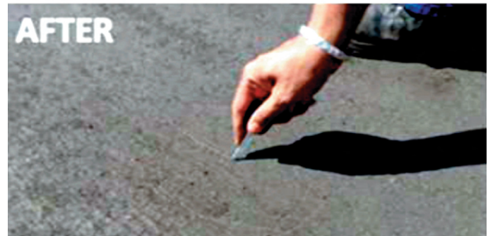
Figure 4. Photographs shows improved road structure and particle bonding after application (courtesy, I-Cat Environmental Solutions, www.i-cat.co.za)
