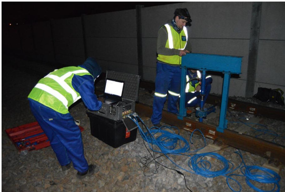
Figure 3.28: Calibration Rig for the Vertical Strain Gauges
