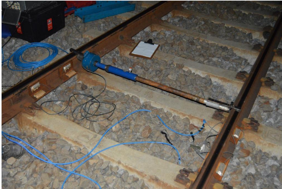
Figure 3.27: Improved Set Up of the Calibration Rig for the Lateral Strain Gauges
