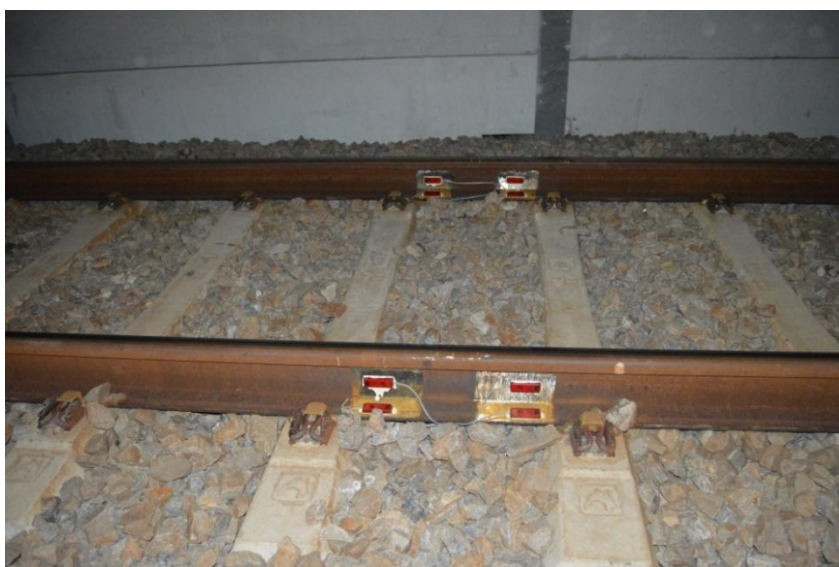
Figure 3.21: Side View of Installed Encapsulated Strain Gauges
