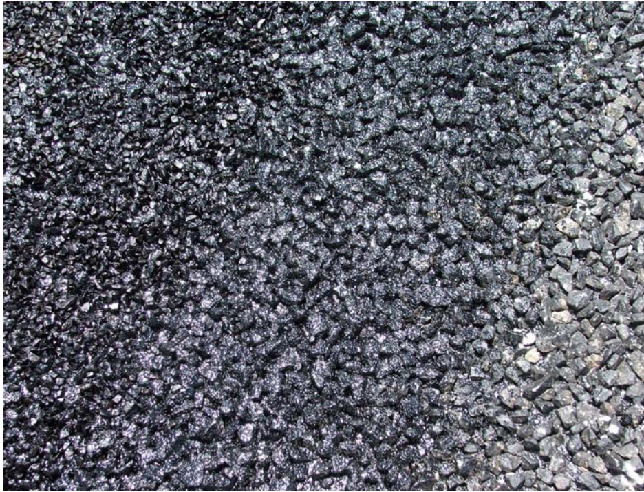
Photo 2: 19mm and 9,5mm double seal (note the stone application rates)
