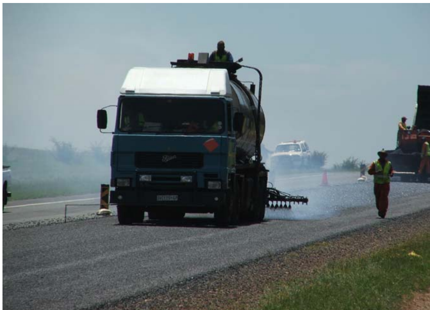
Photo 1: Spraying of Penetration Coat
