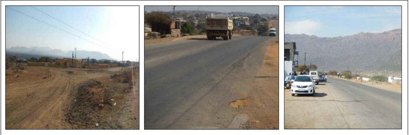
Fig. 3. Existing Road infrastructure and challenges along Link A1 and R555
