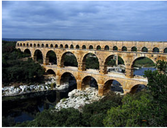
Figure 1. Pont du Gard in Gard, France.
