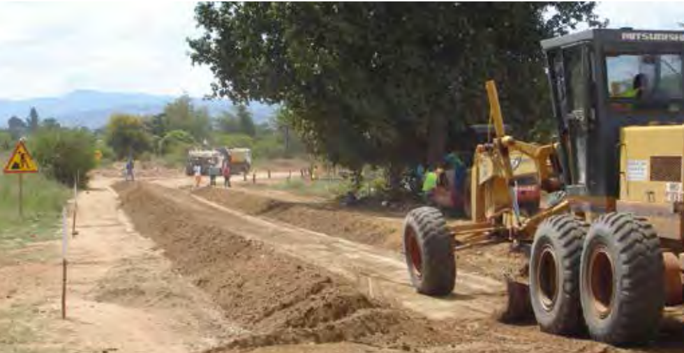
Mixing of nanopolymer-modified emulsion into base layer using conventional equipment
