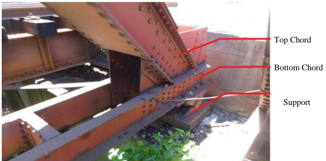
Figure 4.7: Support condition of the actual bridge
