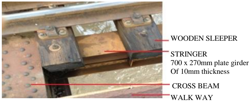
Figure 3.9: Section showing stringer and cross beam
