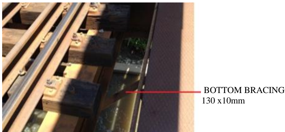
Figure 3.10: Section showing bottom bracing
