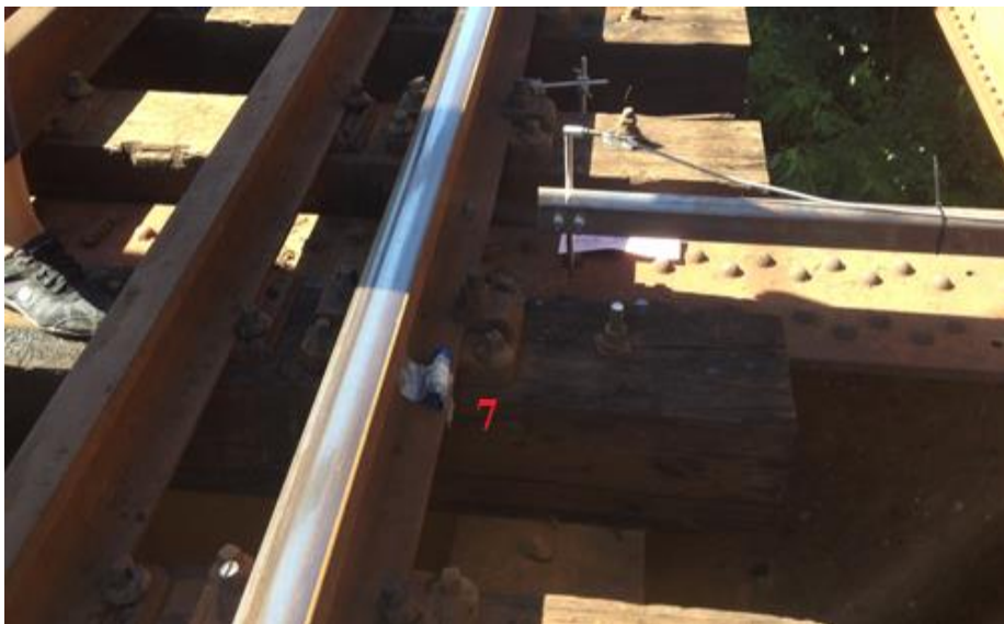
Figure 3.19: Accelerometer fixed at point '7'
