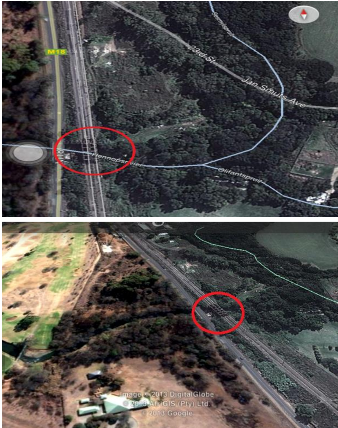
Figure 3.1: Satellite view of the bridge at Irene, Centurion, South Africa
