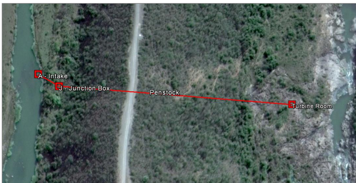
Figure 5-80 - Junction Box and Penstock - Eskweleni SSHP
