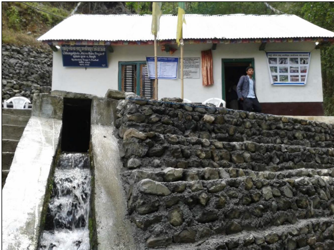
Figure 2-26 - Powerhouse with clear tailrace
