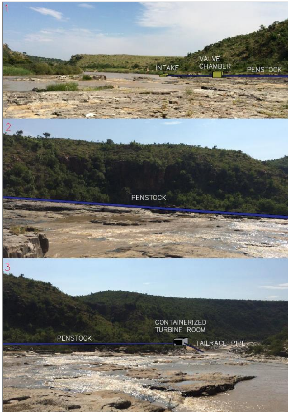
Figure 5-15 - Dunudunu SSHP - Intake and Penstock
