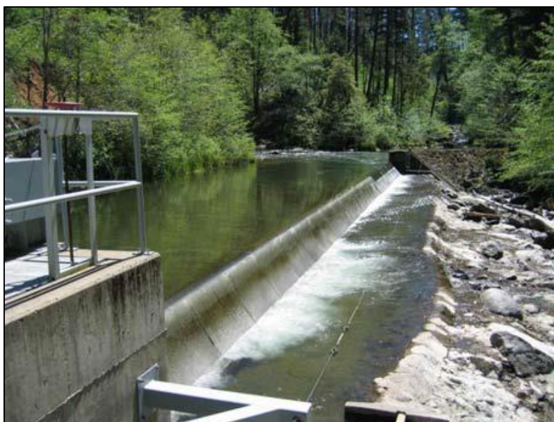
Figure 2-17 - Montgomery Creek intake – Coanda Screen - Shasta County, California, USA (Wahl, 2003)
