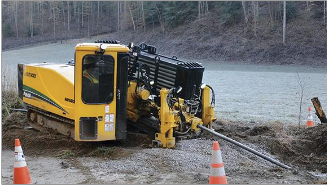
Figure 5-47 - Directional Drilling Equipment (Vermeer)
