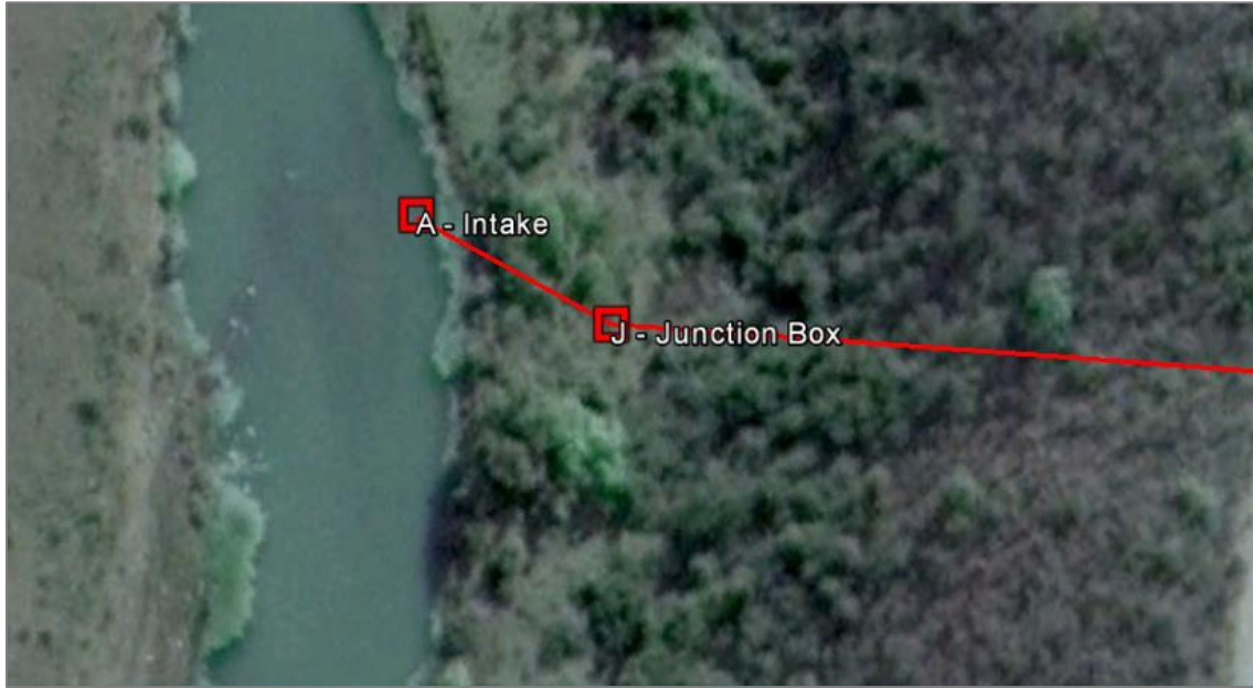
Figure 5-78 - Junction Box - Eskweleni SSHP
