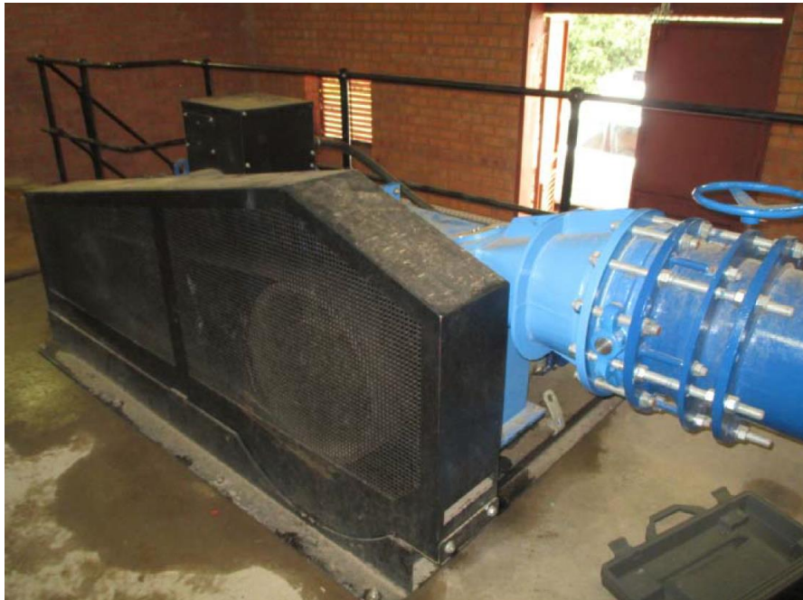
Figure 2-51 - Example of belt driven cross-flow turbine at Bloemwater, Bloemfontein, South Africa
