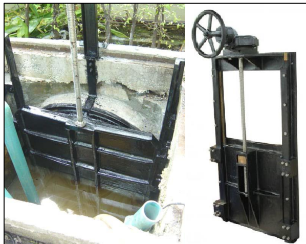
Figure 2-61 - Sluice Control Gate (Penstock) (wemvalves.com)
