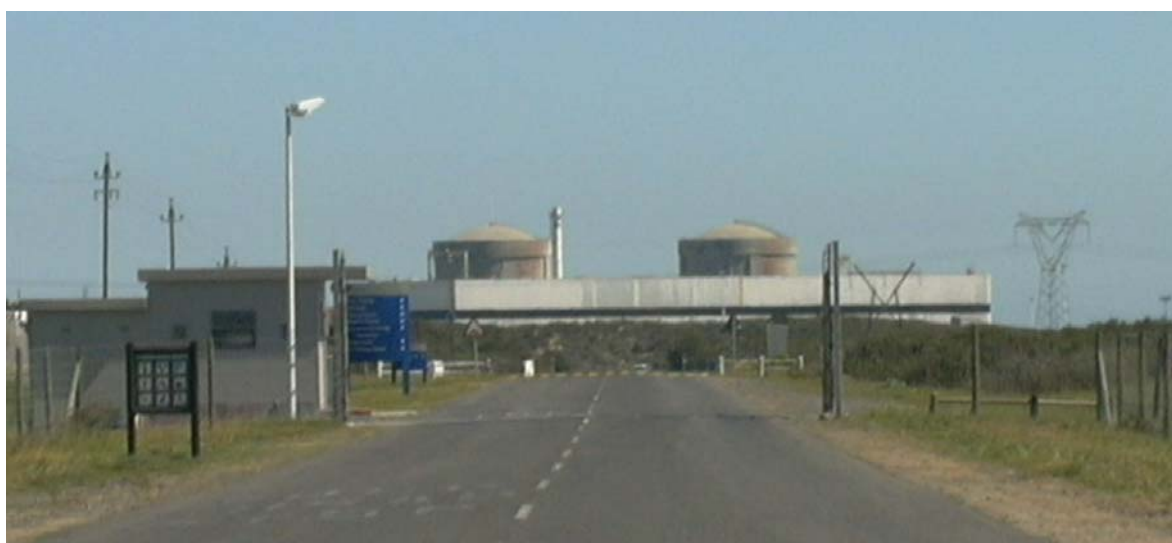
Figure 6. Koeberg Nuclear Power Station.
