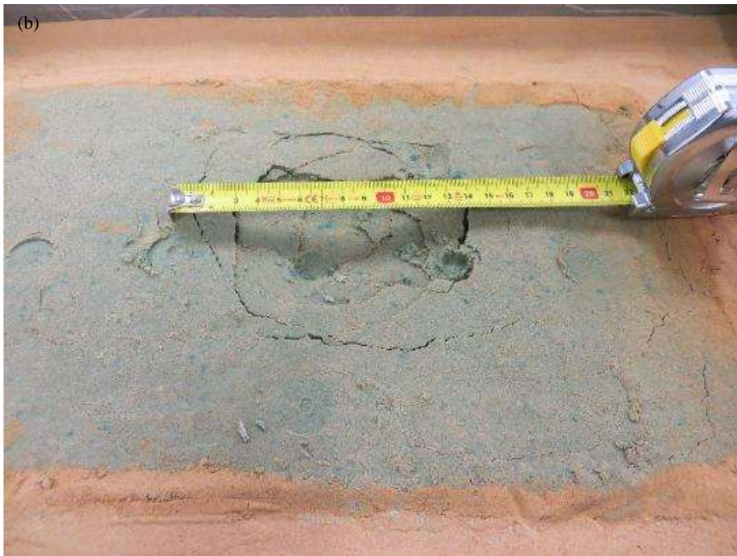
Fig. 6 Comparison of sinkhole related damage to the unreinforced (a) and reinforced (b) soil mattresses respectively.
