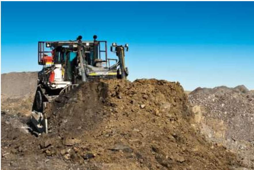
Picture: Photo of a bulldozer at work at the Isibonelo Colliery.
