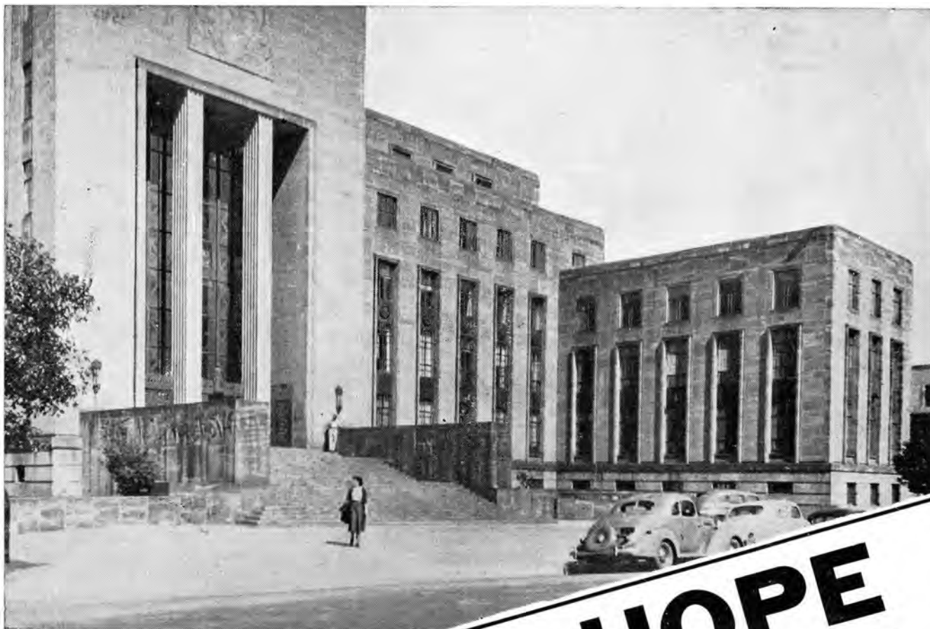
Anglo-American Building, Johannesburg
