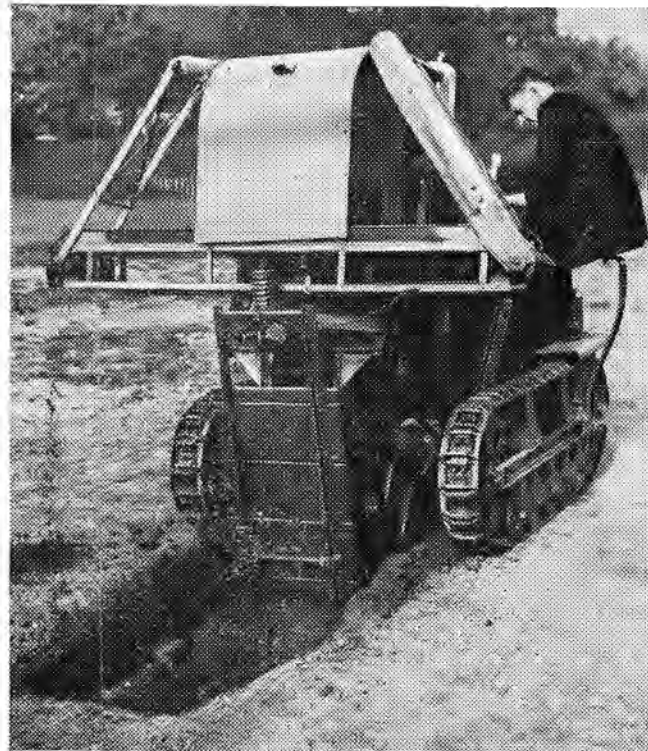
New British machine for building operations, designed primarily for excavating house footings.
