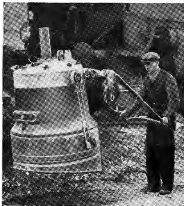
A new type of rammer for straightening weak foundations like unstable clay soil.
