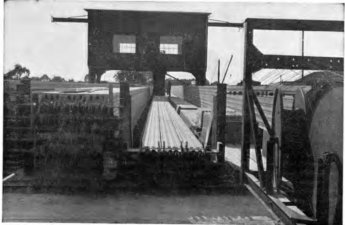
General view of casting bank and mixing machine for pre-stressed concrete in Germany.
