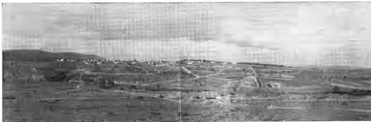
View of the Rooikrantz Dam site from the right flank (towards the right centre of the picture). The construction camp is in the background.
