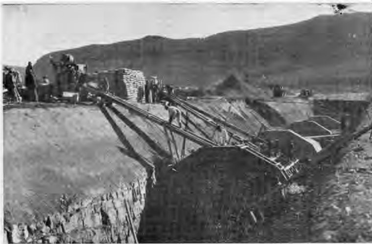
View of outlet culvert through the dam, under construction.
