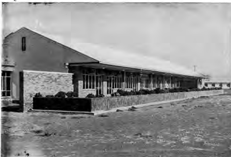
View showing back of wards on north front, with the nurses' home in the background.
