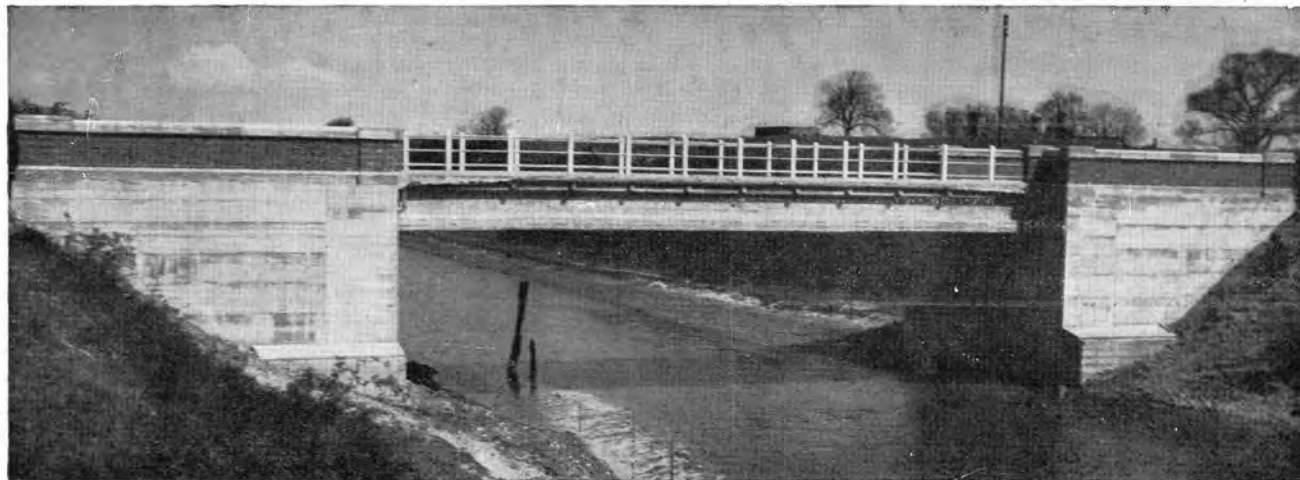
Above : Pre-stressed in situ concrete bridge at Fishtoft, near Boston, Lincs.
