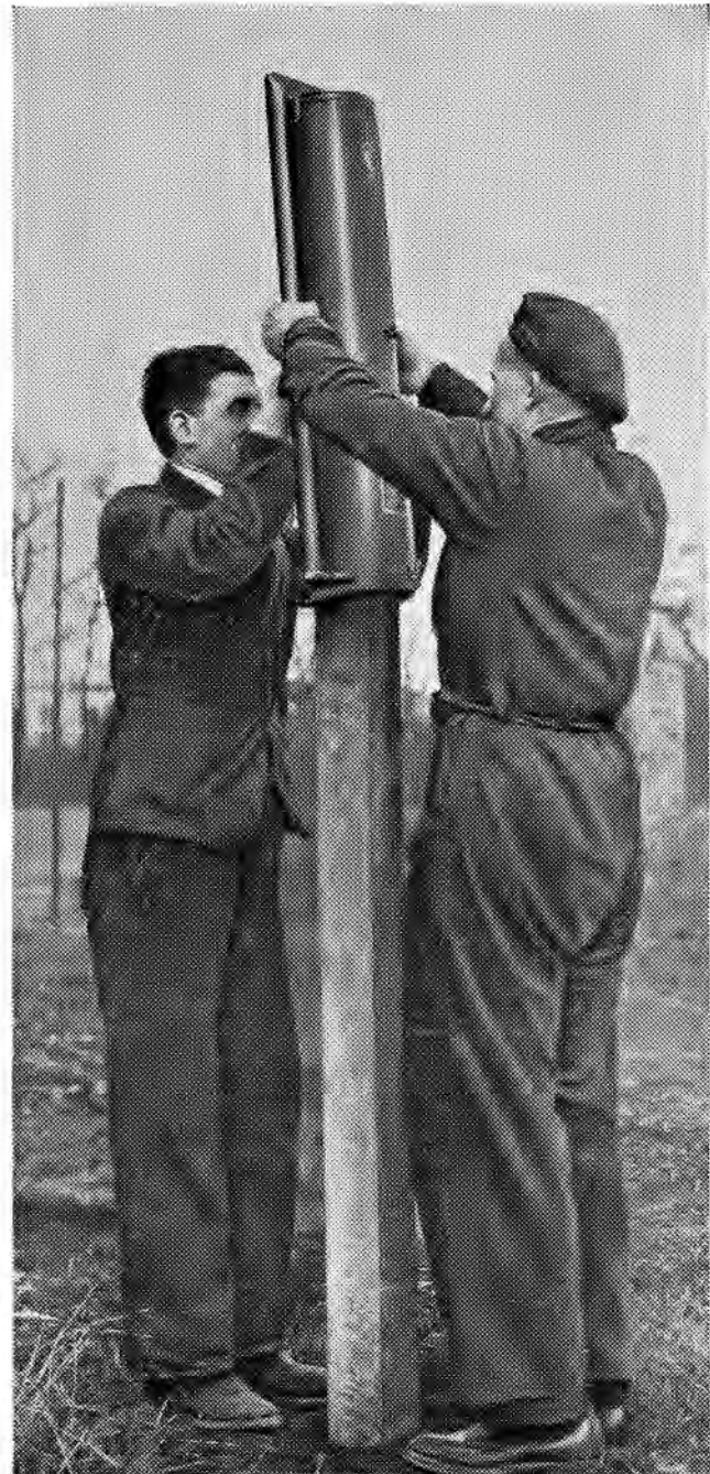
New British stake-driving tool, which enables two men to put in the ground nine stakes in five minutes — more than they could manage in an hour with the usual spade and rammer.
