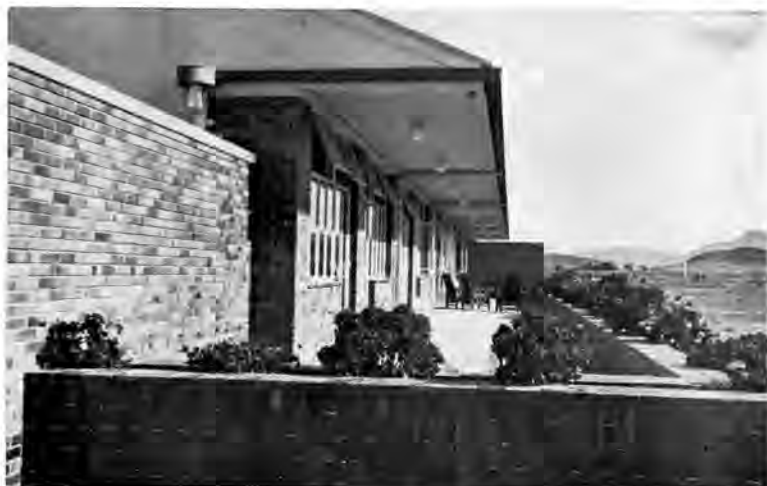
North terrace in front of the wards, showing eave projections and Coloured verandah in foreground.
