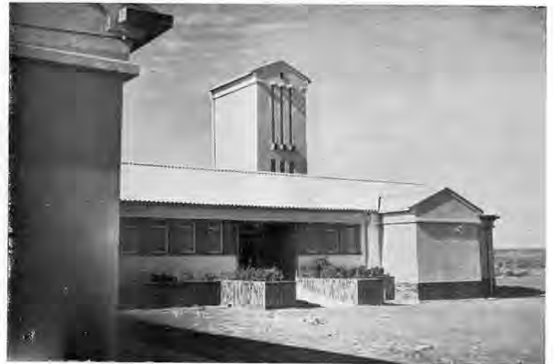
Main entrance to building, showing water tower containing supply tanks and water softening plants.
