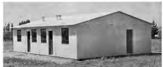
Photo No. 5. Block of completed houses with concrete slab roof.
