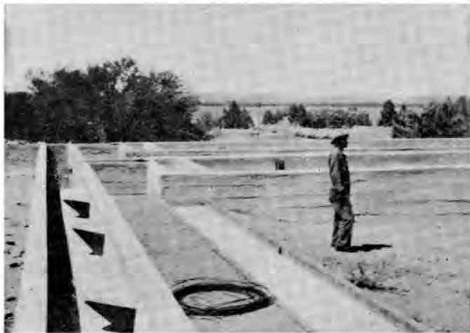
The mixing channel from the dosing house to the sedimentation tanks.
