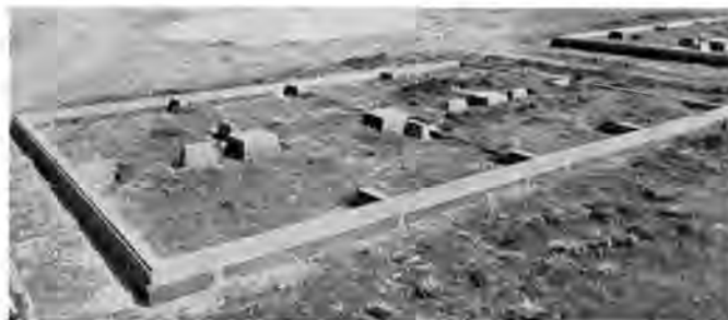
Photo No. 1. Foundations and underbuilding complete.
