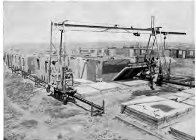
Photo No. 4. Wall panels being erected by special gantry.
