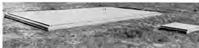
Photo No. 2. Floor slab cast.
