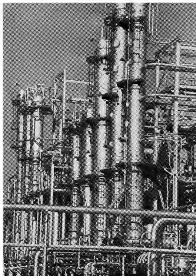
The hydrocarbon or fractionating unit of the new Stanlow chemicals plant, which will manufacture solvents previously obtained for Britain only from dollar sources
