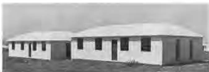
Photo No. 6. Block of completed houses with cast in-situ concrete shell roof.
