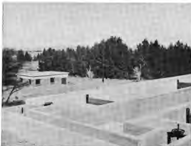
Entrance to the sedimentation tanks from the mixing channel.
