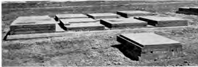
Photo No. 3. Wall panel cast in layers, ready for erection.
