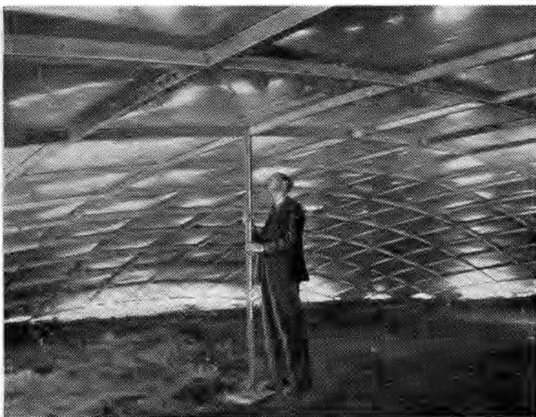
A new type of roof, made of aluminium, was shown at the recent British Industries Fair. With an 83-ft. diameter and a centre rise of 9 ft., six men can erect all the framework and weld all the shoes, down to the outer support ring, in a day.
