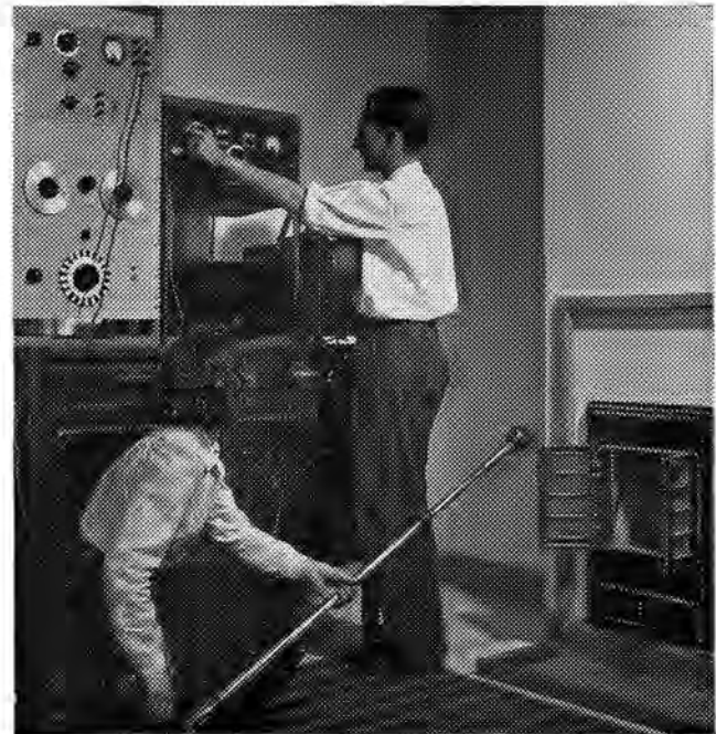
Experiments on house-heating carried out by technicians of the Department of Scientific and Industrial Research at Abbot's Langley, Hertfordshire. The picture shows electric equipment to measure the amount of noise in the heat ducts in the walls.
