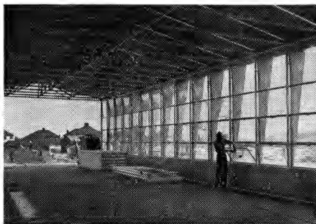
Five aluminium schools are being built by the Kent County Council. This view depicts one of the six main classrooms at St. Paul's Cray, Orpington.
