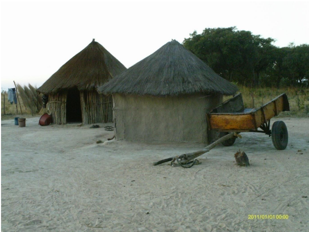
Figure 8: A photograph taken showing poor home infrastructure
