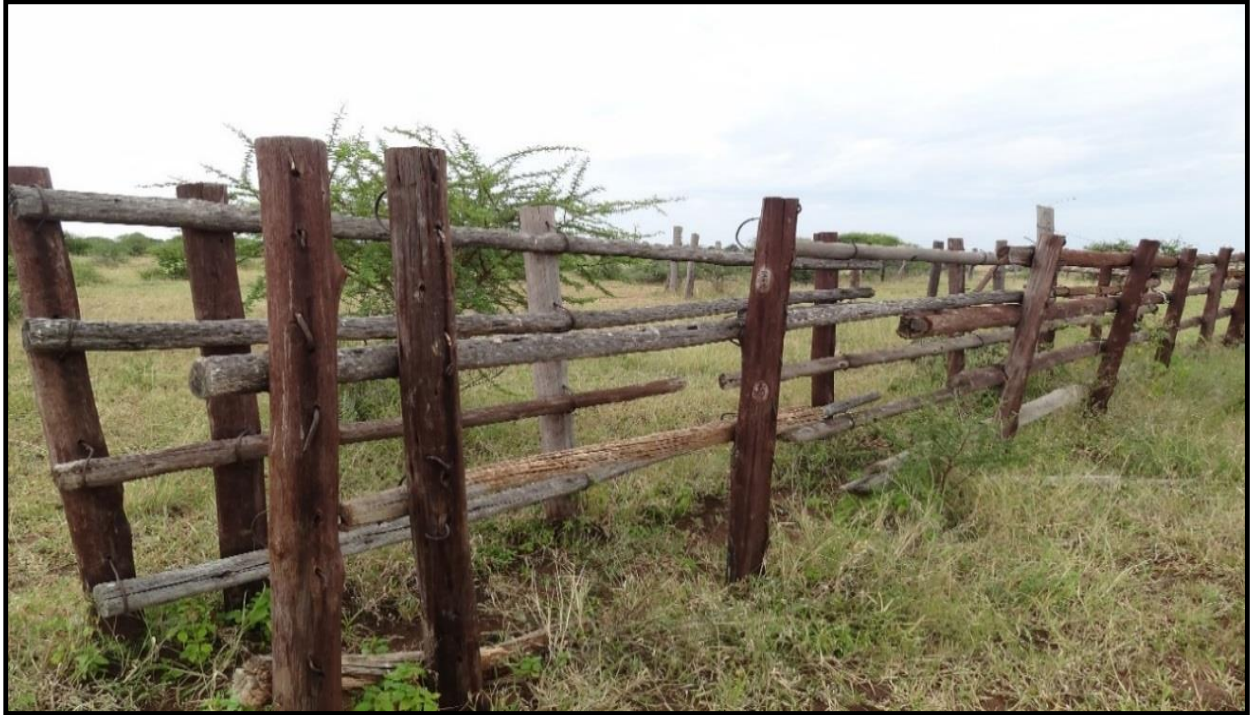
Figure 3.4 One example of the dilapidated crush pen in Mootla village
