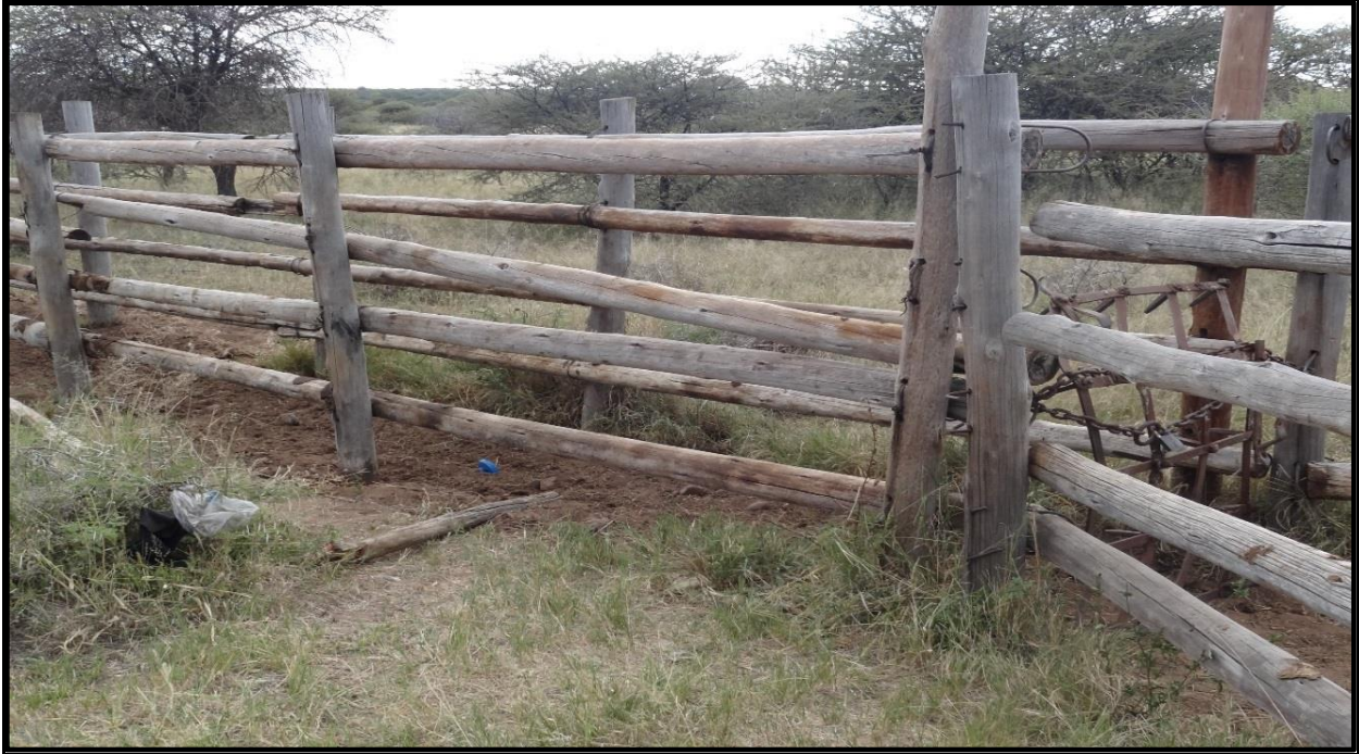
Figure 3.6 Dilapidated crush pen at Sutelong village
