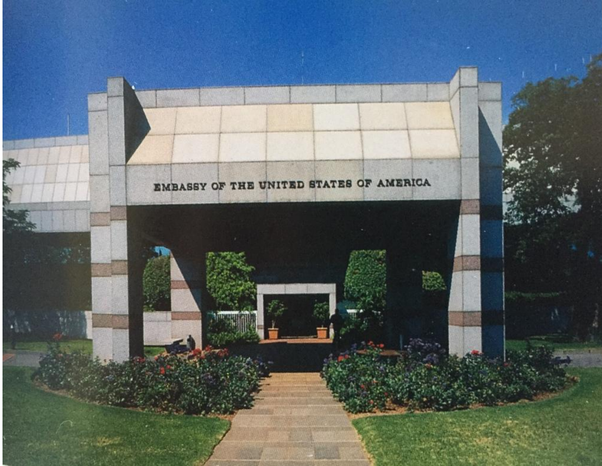
Image 4.1: U.S. Embassy, Arcadia, City of Tshwane (Main entrance) Photograph taken by Elizabeth G. Lui In (2004) Building diplomacy... p 41
