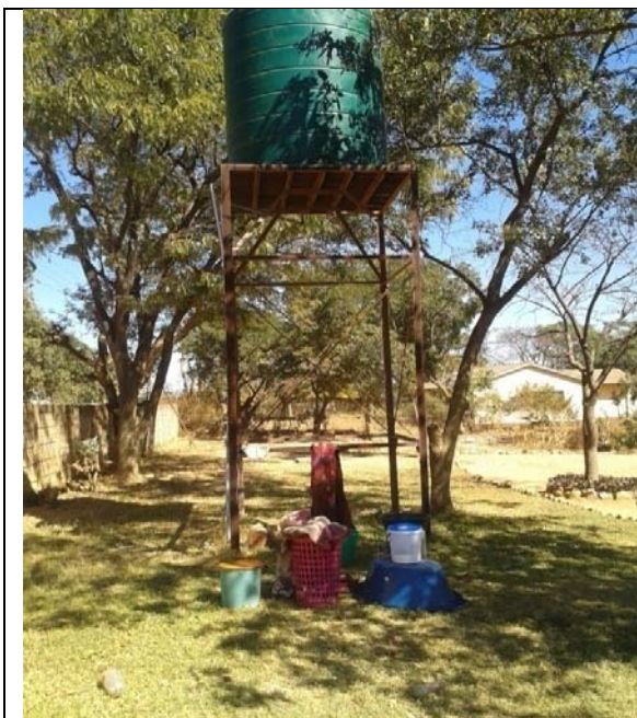
Fig 8: Typical storage tank of household boreholes water in the LDSs.
