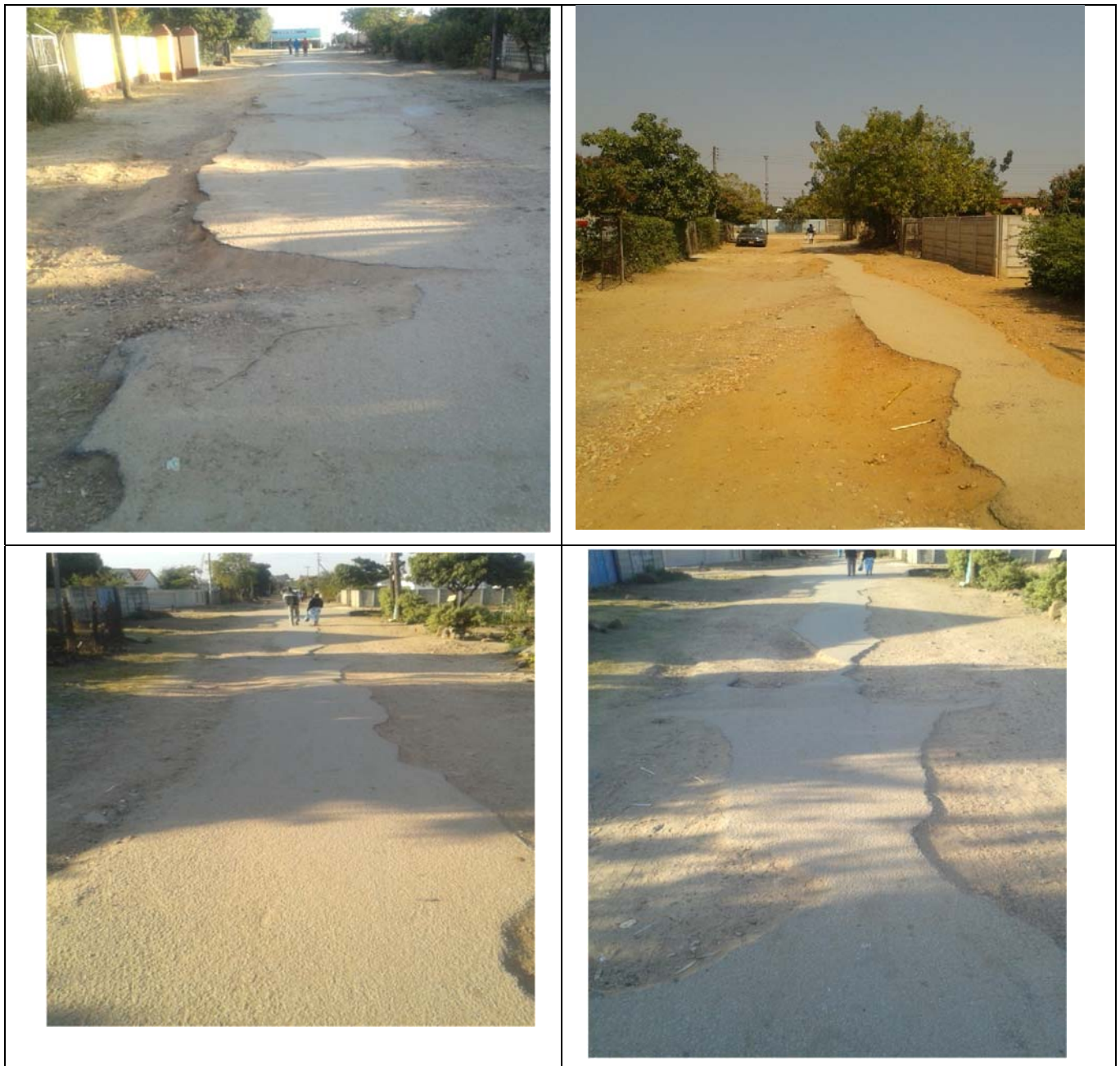
Fig 6: Roads in High Density Suburbs (HDSs)
