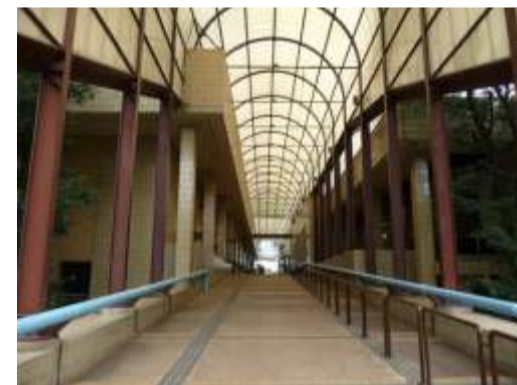
Figure 2.5.3.2. Ramped walkway to entrance.
