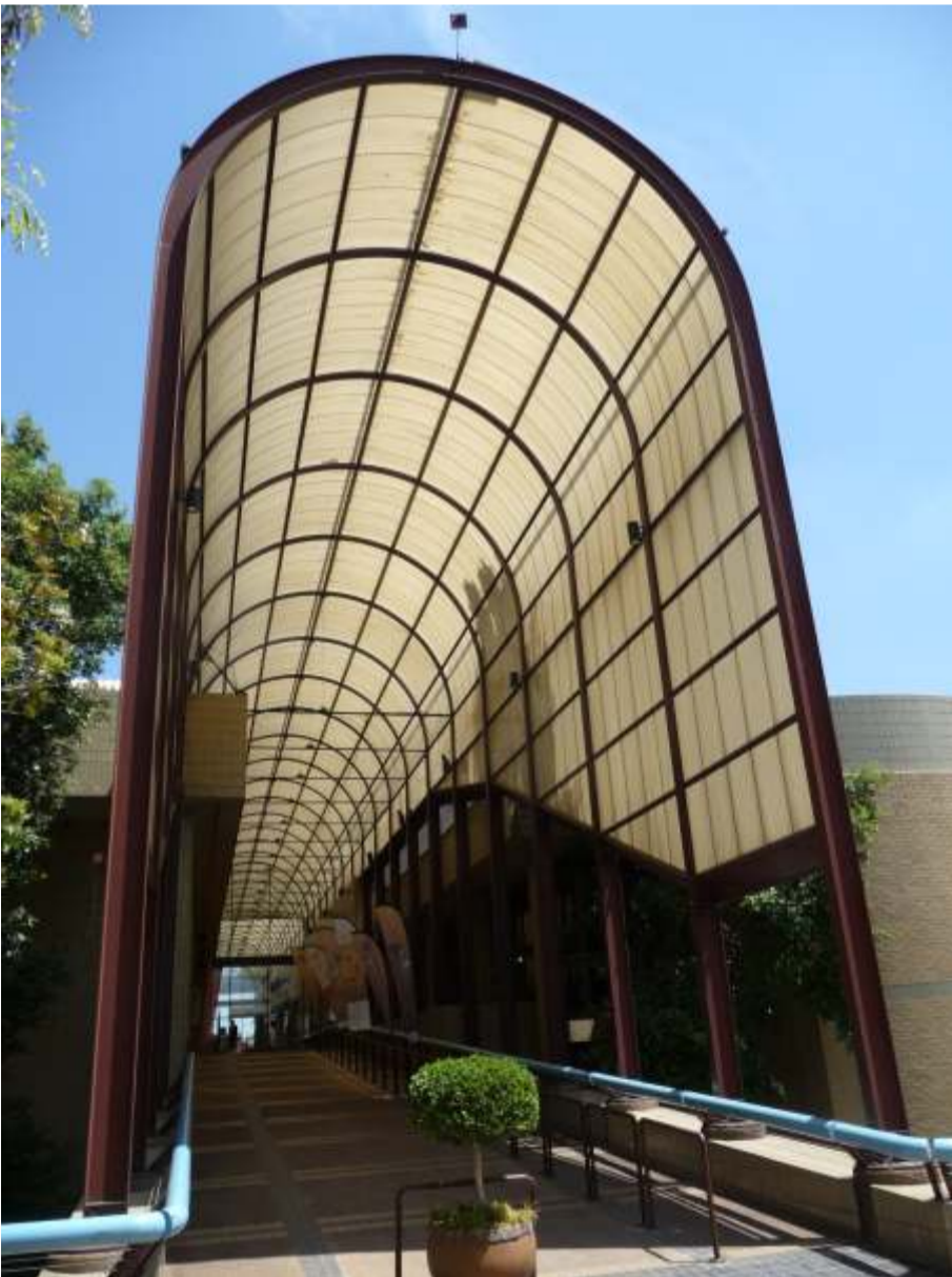
Figure 1.1.1. Ramped walkway to main entrance of the Ditsong: National Museum of Cultural History.
