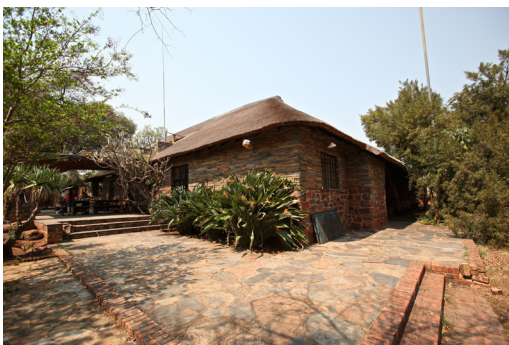
Figure 09.04: The Preller House in Pelindaba, Hartbeespoort dam
