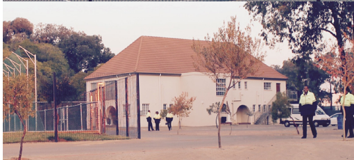
Figure 03.24: Tennis house - heritage protected buildings on PHSG's grounds, viewed from Loftus' current grounds (photographs taken by Author, 2015)
