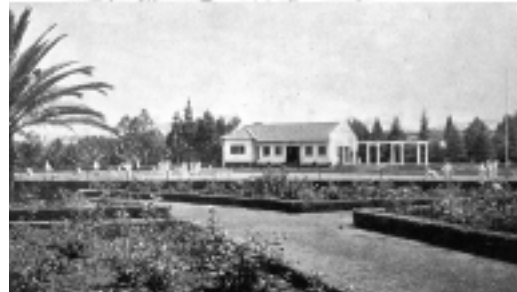
Figure 03.45: The pergola that extended from the eastern facade and original garden (Coetzee, 2012)
