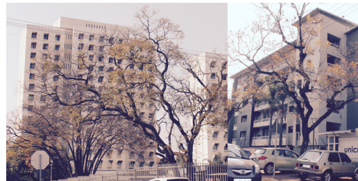
Figure 03.18: High rise student residential buildings in Hatfield (Author, 2015)
