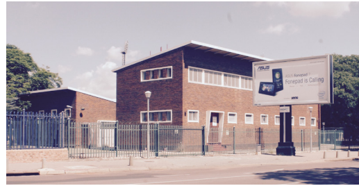
Figure 03.50: Loftus Substation - view from Kirkness street (Photograph taken by Author, 2015)
