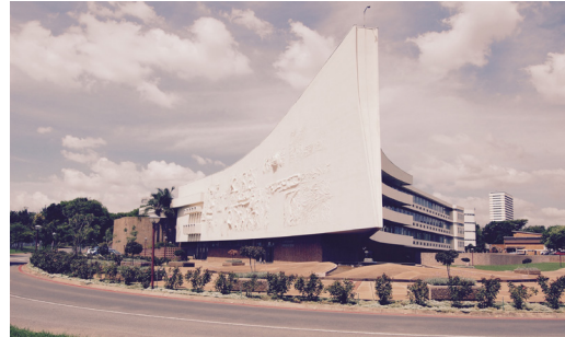
Figure 03.23: The Ship (Administration Building) at the University of Pretoria, situated on the corner of Lynnwood and University Streets
