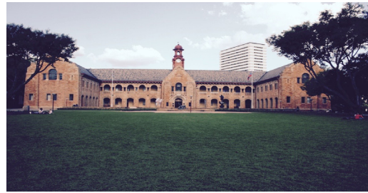
Figure 03.22: The Old Arts Building at the University of Pretoria (to which the historical line of trees line up with)
