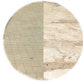
Brick Paving and Concrete
