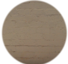
Concrete Brick Walls
