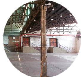
Timber and Steel Column
