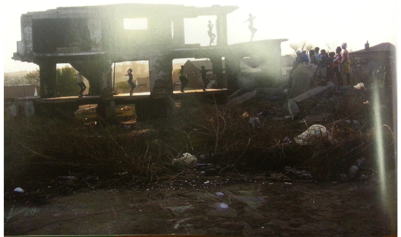
FIGURE 86 - THE SANS SOUCI: BEFORE INTERVENTION (LINDSAY BREMNER ARCHITECT & 26'10 SOUTH ARCHITECTS)
