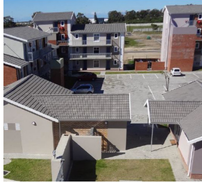
Figure 6.20 Walmer Link, a housing scheme divided into two developments: Social Rental and Affordable Housing to also provide for the gap market. The project is financed by the Finance Linked Individual Subsidy Projects (FILPS) (GM South Africa Foundation).
