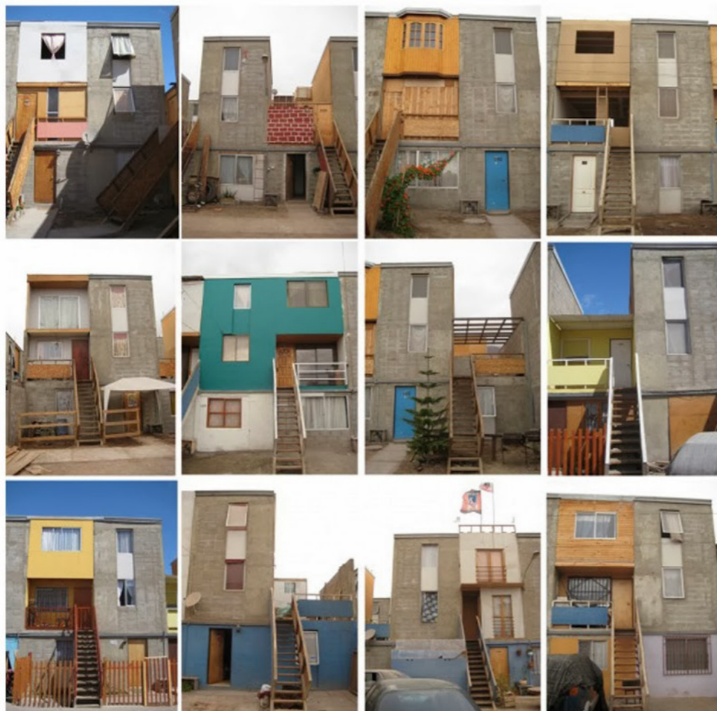
Figure 6.2 Quinta Monroy after occupant alterations (Aravena, 2013)
