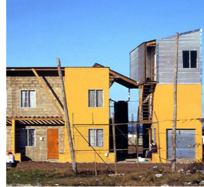
Figure 6.22 Pelip Housing, Red Location, Port Elizabeth. Despite the political situation and initial conflict with local communities against the unconventional housing project, the project set out to challenge the government approach - that is to provide a free-standing house for every family in South Africa (Noero 1999:29)
