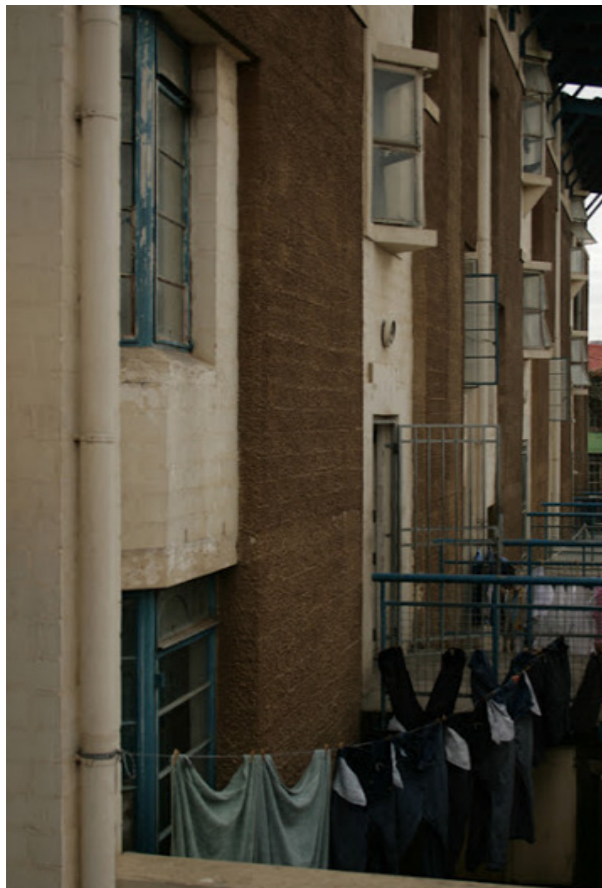
Figure 6.26 Units with laundry space in backyard (Wolff)
