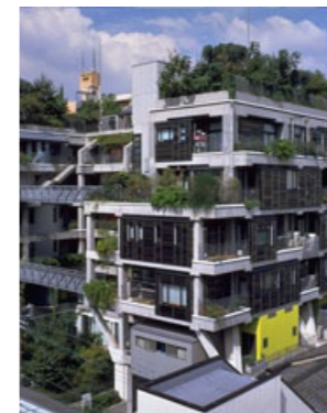
Figure 6.4 Next 21, Osaka, Japan with a permanent infrastructure with the infill having a shorter lifespan is designed to be easily replaced (Kendell & Teicher, 2000)
