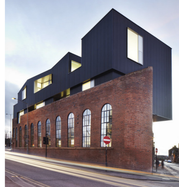
Figure 6.32 After completion (Sheffield 2012)
