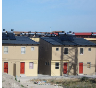
Figure 6.21 N2 Gateway Project is located in Joe Slovo (Langa, Cape Town) demonstrating new ways of developing human settlements with social and economic amenities along with housing units (Tonkin, 2008)
