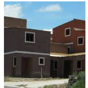
Figure 6.6 K206 in Alexandra, Johannesburg, a second local example of open building (CSIR, 2011)
