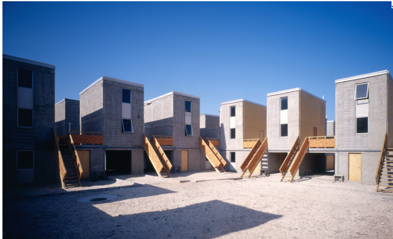
Figure 6.1 Completed housing unit before occupant alterations (Elemental, 2008)
