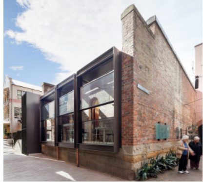
Figure 6.28 Former Rocks Police Station with a new steel and glass to accommodate its new use as a café (Acorn 2014)
