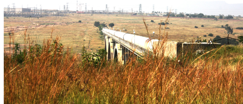
Figure 53. view of sewage pipe with power plant in the background (Author 2015).
