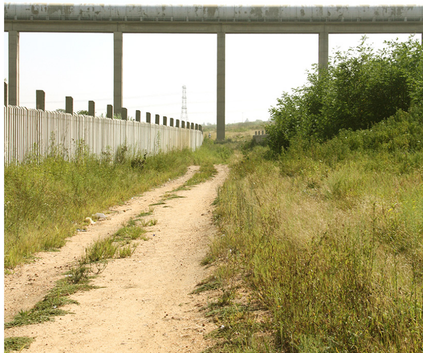
Figure 40. Sewage Line as seen from within an informal road on the DNR (Author 2015).
