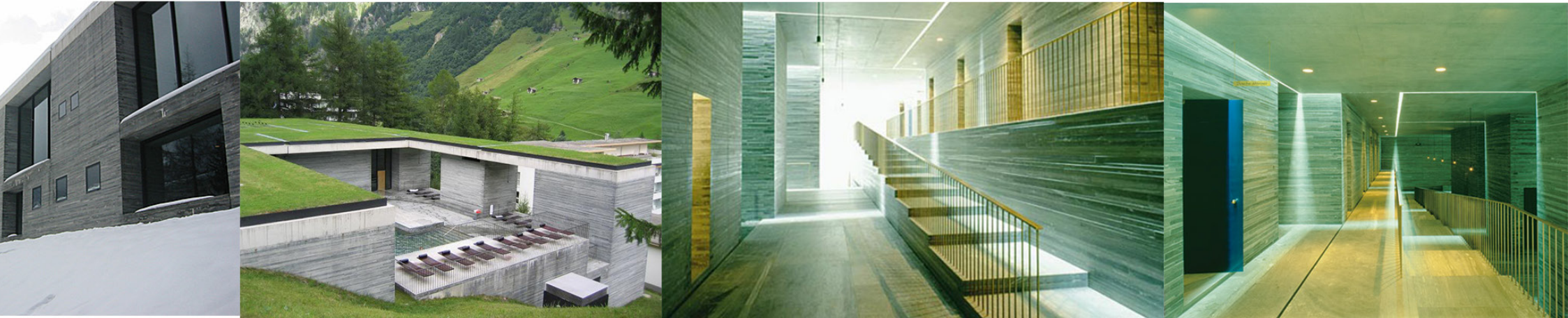
Figure 124. Thermal baths, Switzerland, by Peter Zumthor. Spaces are created through carving it from a solid structure (Betsky 2002).
