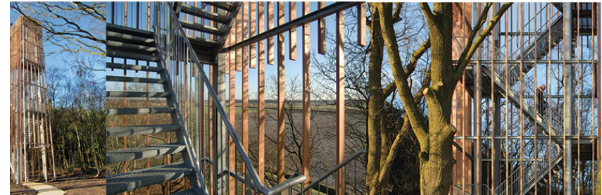
Figure 122. Tectonic viewing tower at Vecht riverbank in Dalfsen (Author 2015).
