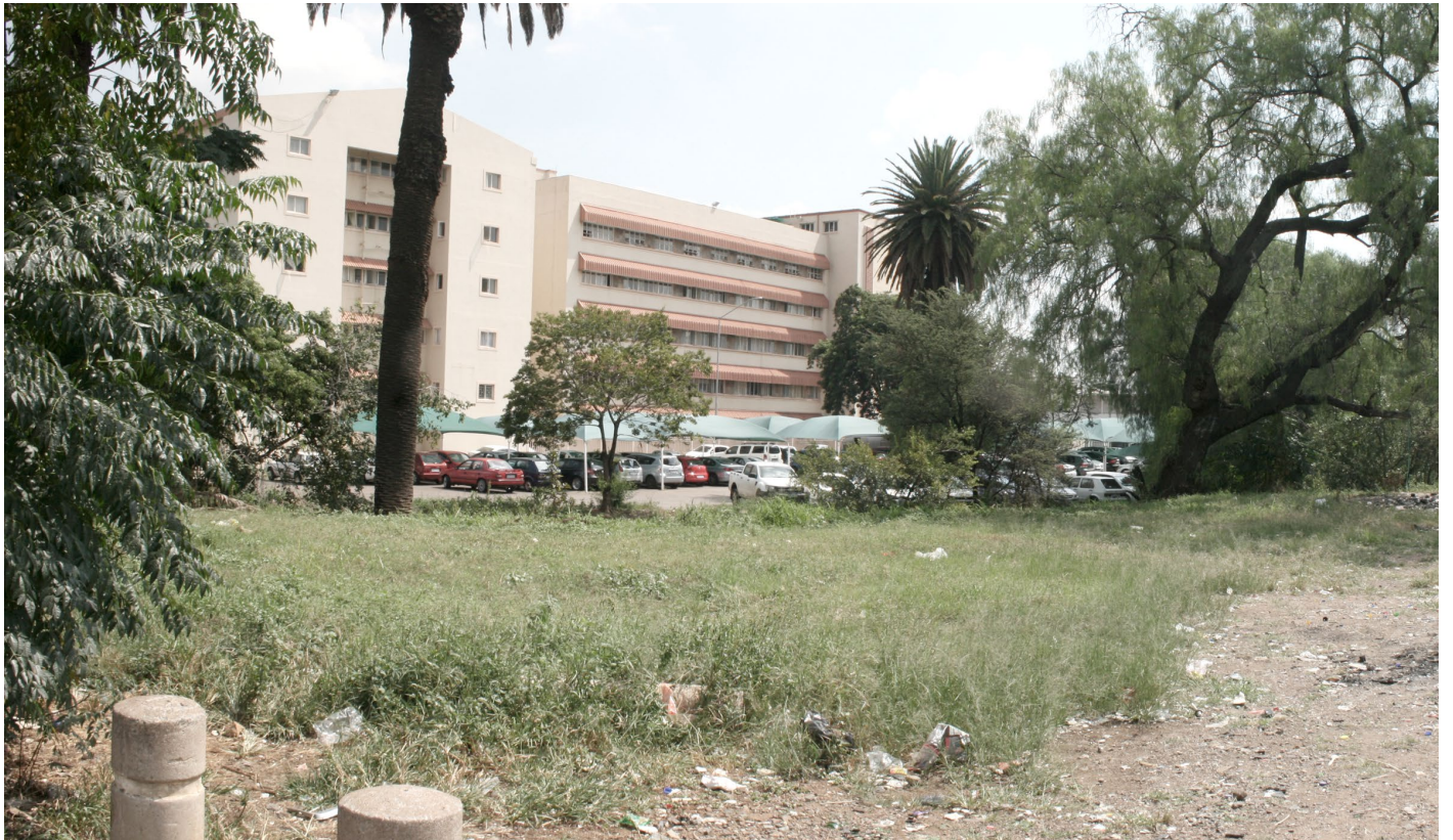
Figure 5.7: Panoramic view from Pretorius Street onwards the site. (Photograph by Author 2015)
