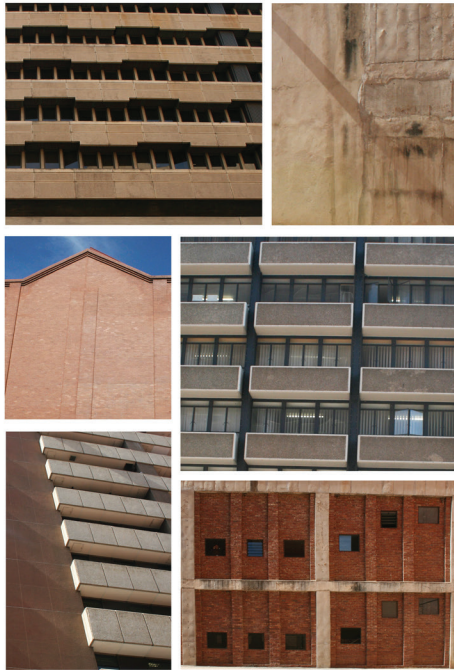
Figure 9.6 Existing Materiality. (Source: Author)
