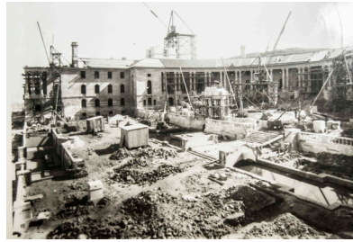
Figure 6.3 Historical images of construction process (National archives)
