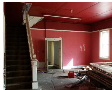
Figure 5.45 Existing staircase to first floor
