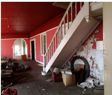
Figure 5.43 Existing staircase to first floor
