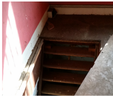
Figure 5.44 Existing trap-door to basement
