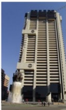
Absa Building 320 Lillian Ngoyi Street Erf 2909/1
