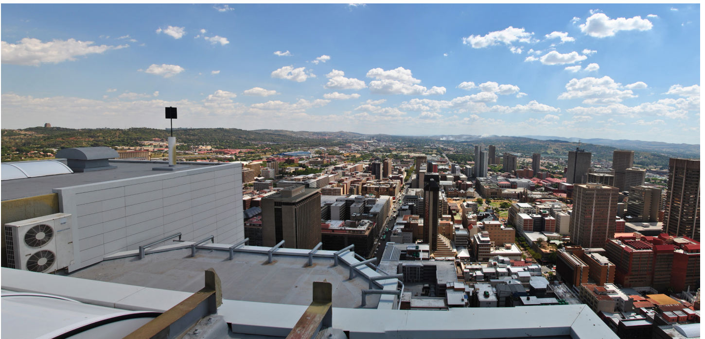
View looking West on top of ABSA Tower
