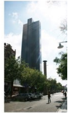
Reserve Bank 370 Church Street Erf 3271
