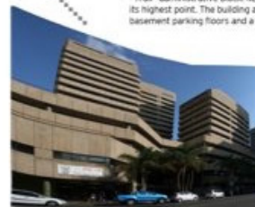
Momentum Building 329 Pretorius Street
