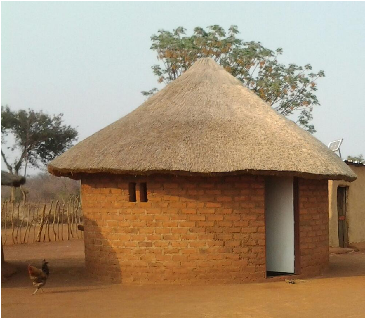
Figure 4.6 Picture of thatched roof of round hut from Chikwanda district
