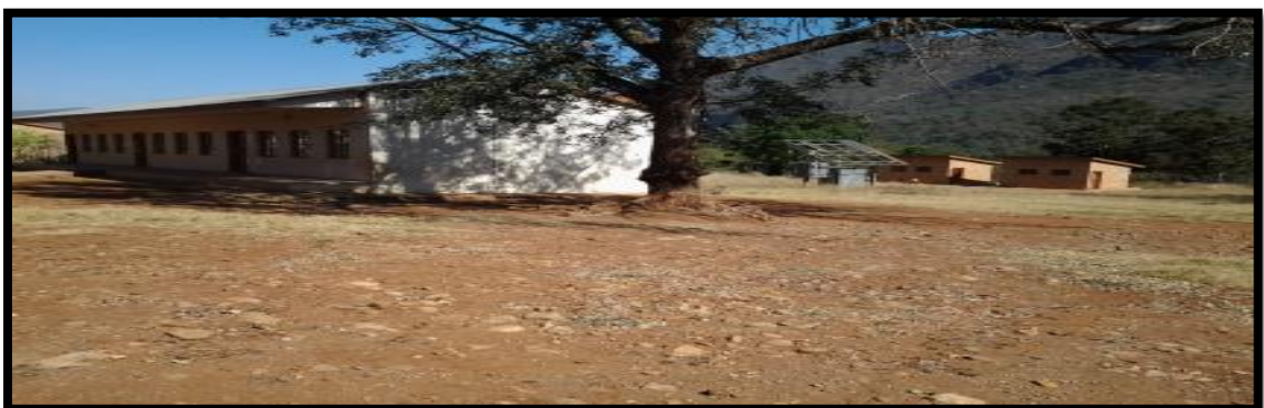
Photo 11: Old block of 3 classrooms at School B
