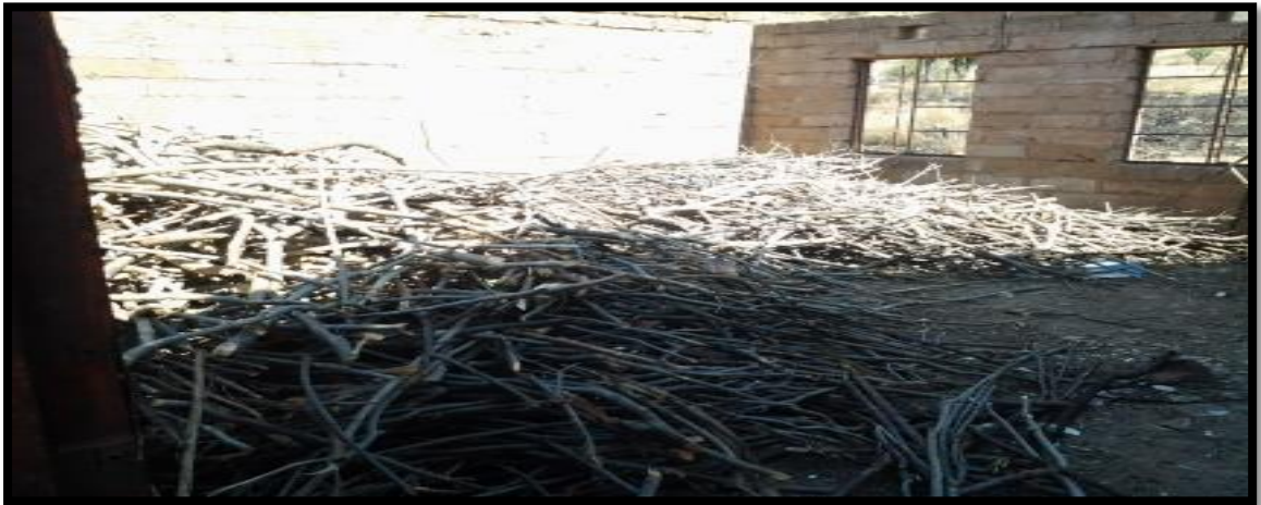
Photo 8: Firewood in one of the dilapidated classrooms
