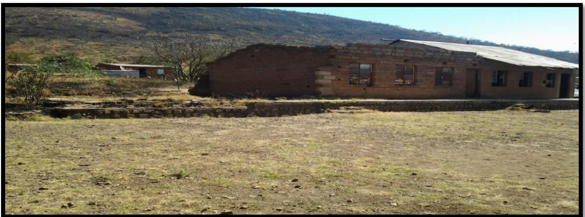
Photo 6: Old block of classrooms with make shift kitchen
