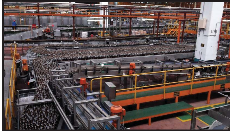
Figure 17: A Section of Conveyer in Process Area 5 that can be Redesigned
