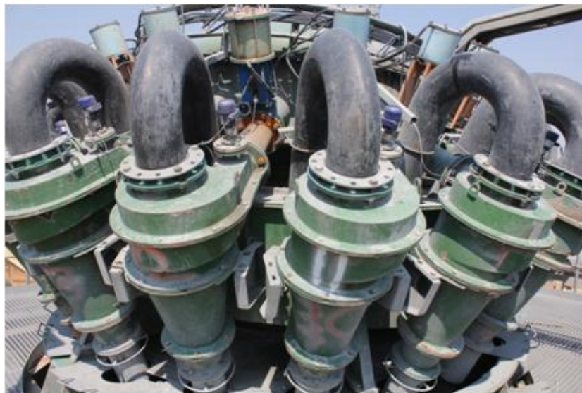
Figure 11: Cyclone cluster utilised as classification stage at Nkomati concentrator plant
