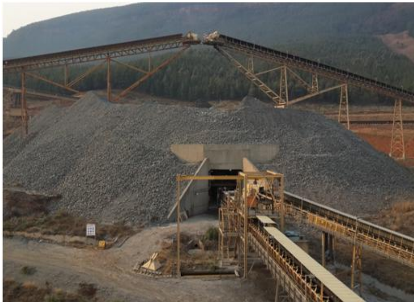
Figure 8: Stockpile of material prior to feeding concentrator plant
