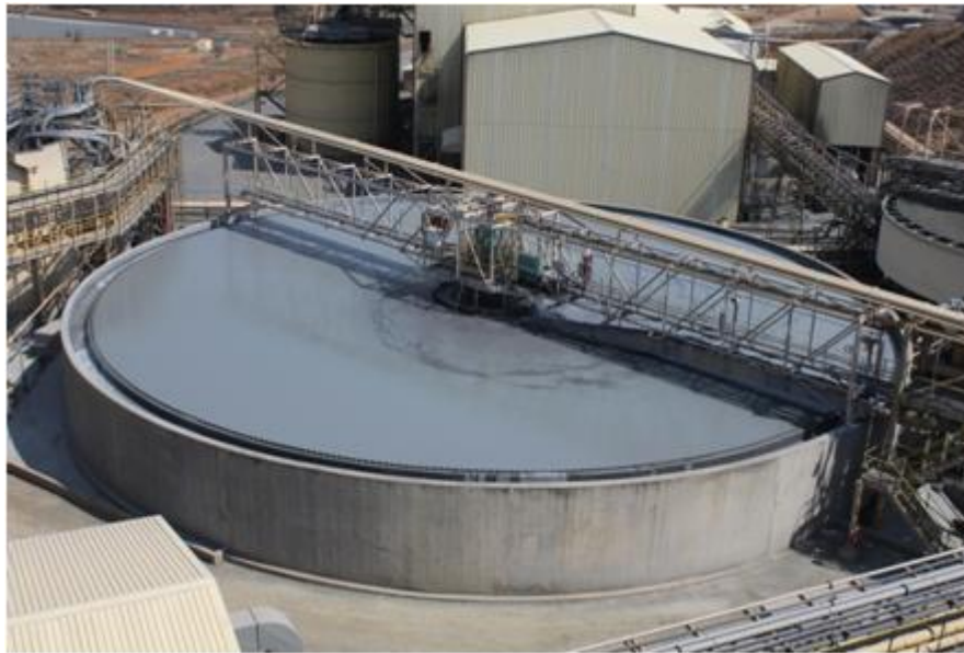
Figure 16: Tailings thickener utilised for dewatering of the final tailings or waste stream from the concentrator process
