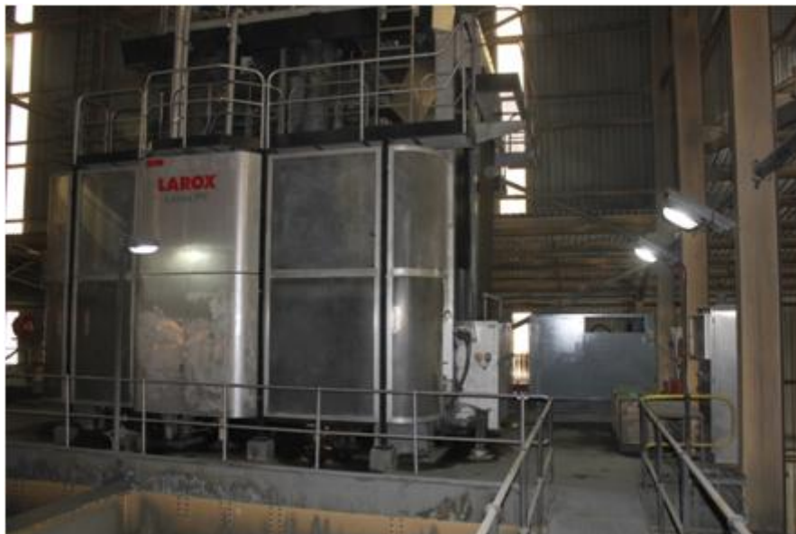
Figure 15: The Larox filter press utilised during the filtration process at Nkomati Mine
