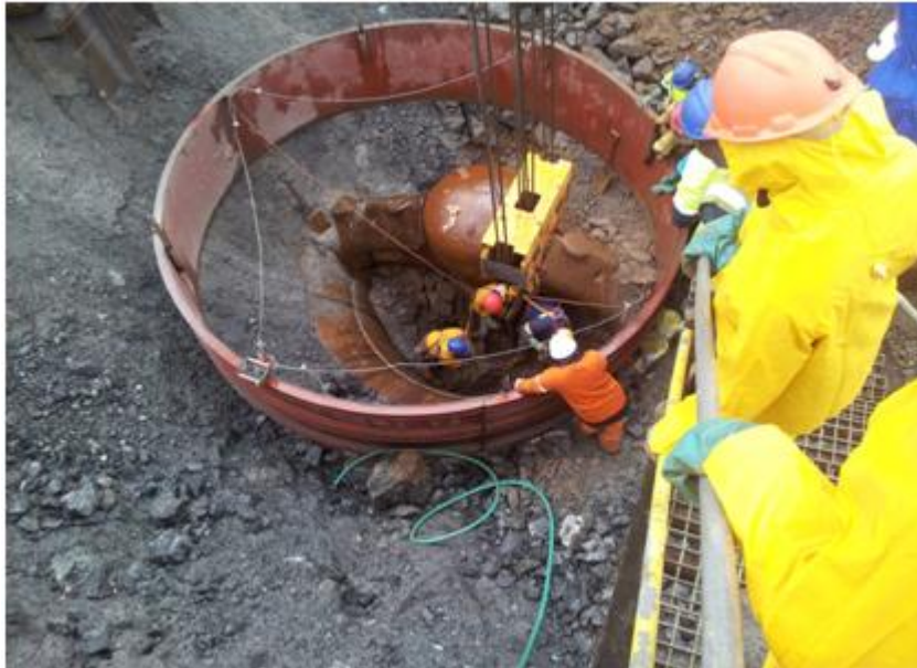
Figure 7: Metso 54" × 75" gyratory crusher used to treat ROM material at Nkomati Mine
