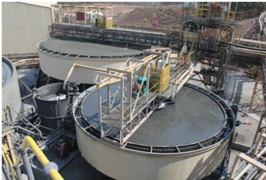
Figure 14: Picture of the concentrate thickener (background) and clarifier (foreground) used to thicken the concentrate produced from the flotation circuit
