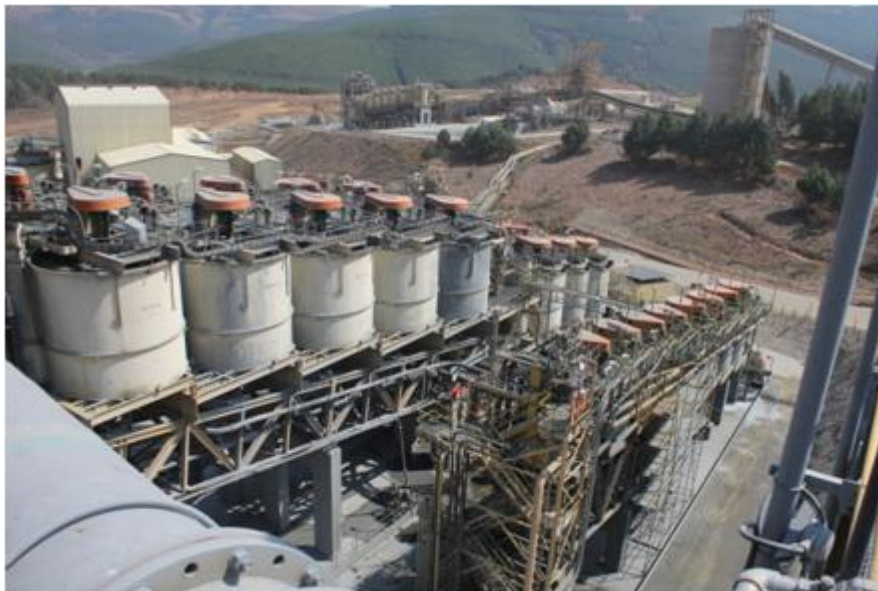
Figure 13: Overview of the flotation circuit utilised in the concentrator plant
