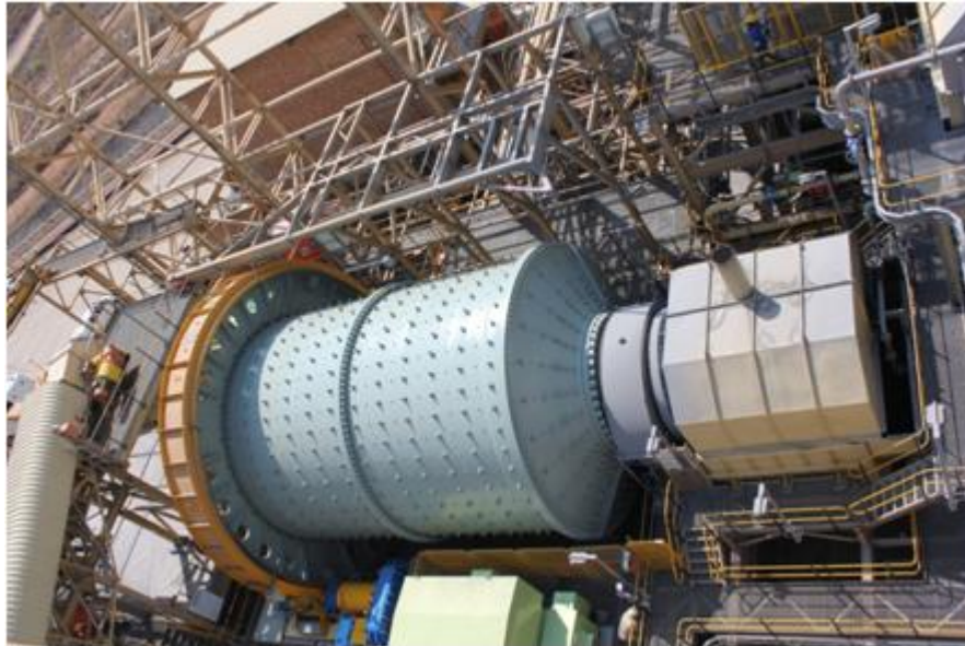
Figure 12: Ball mill utilised for the secondary grinding stage of the Nkomati concentrator plant
