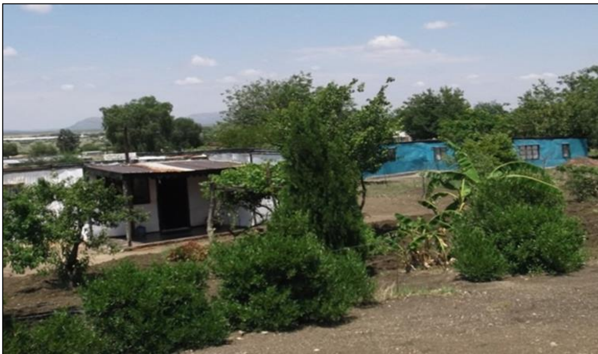
Figure 8: Houses built from metal products as an alternative to the traditional building material (bricks and cement). Note the dark coloured soils associated with expansion.
