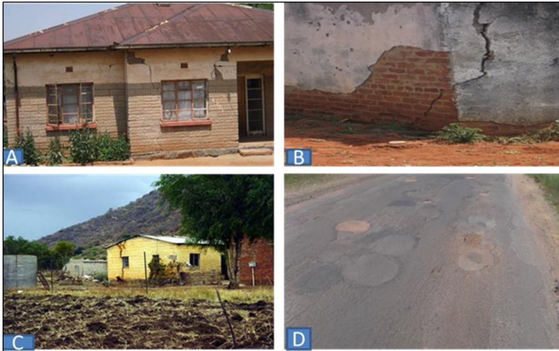
Figure 7: Images from the study area displaying damaged infrastructure associated with expansive soils (image C was taken from CGS archives).
