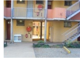
Walkways and/or stairs
