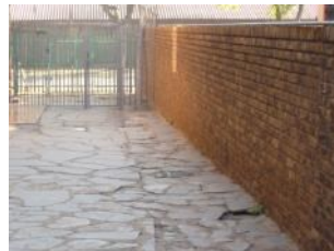
Figure 5.46 Images of the condition of Litakoemi's boundary walls
