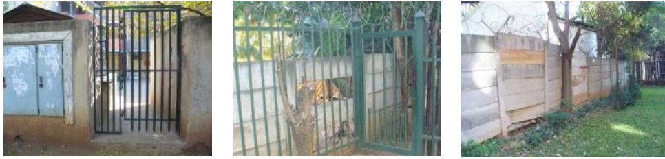
Figure 5.29 Images showing Kopanong’s entrance, northern and western boundary wall
