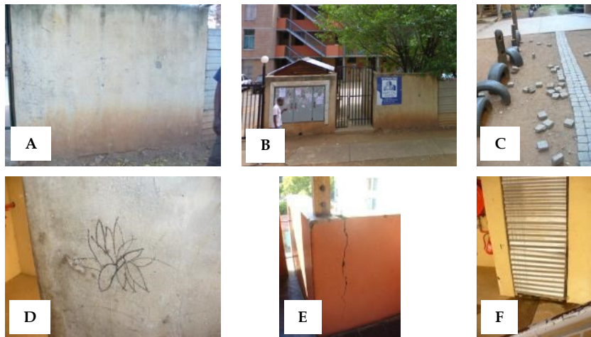
Figure 5.30 Elements that require repair in Kopanong
