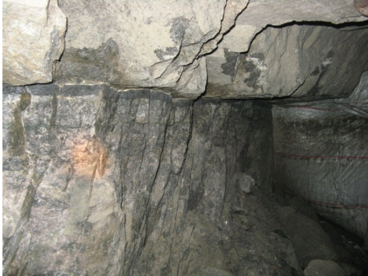
Figure 1-3: Scaling facilitated by a weak contact at the pillar/hanging wall contact
