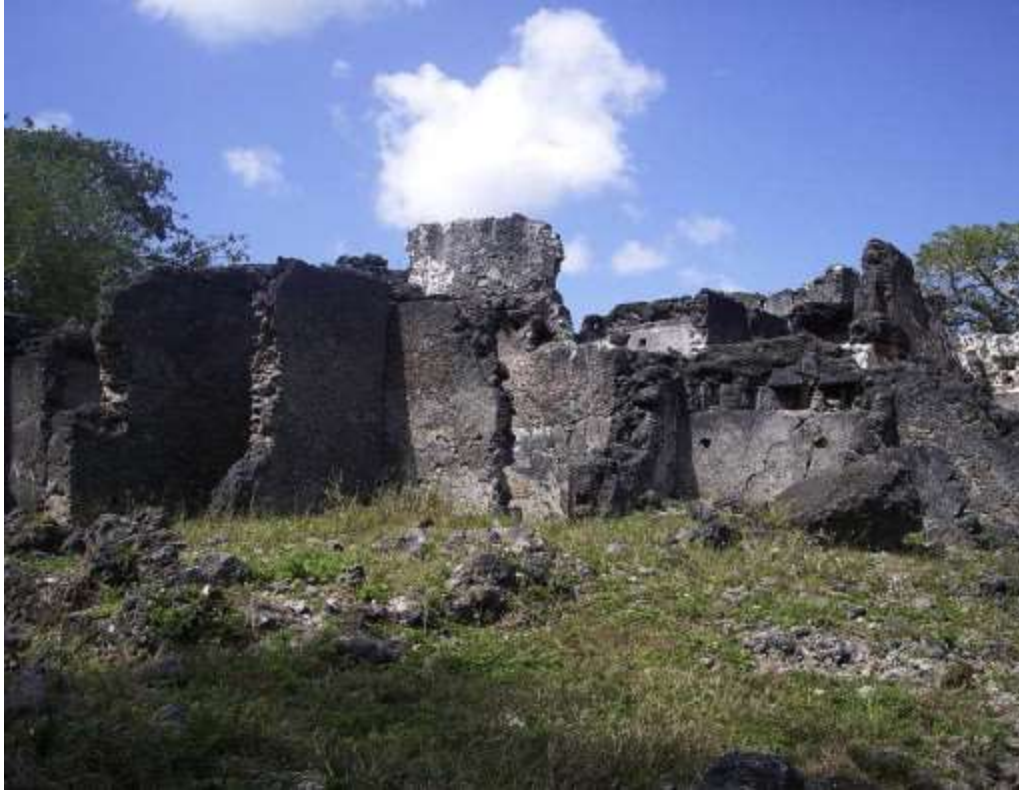
Fig. 3: Standing architecture at SM
